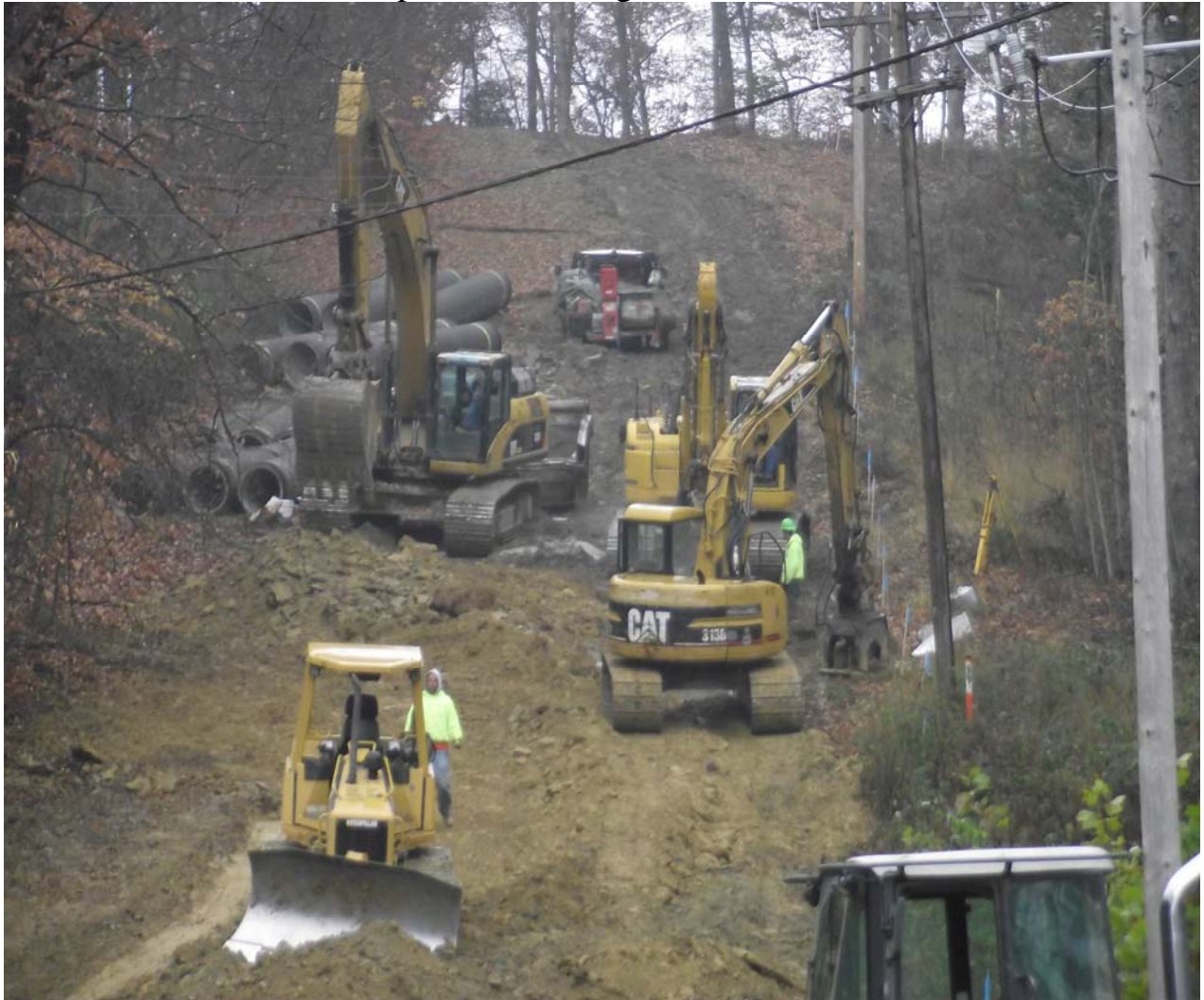
4.5.3.3. Installation of Fire Line Revised August 6, 2014
