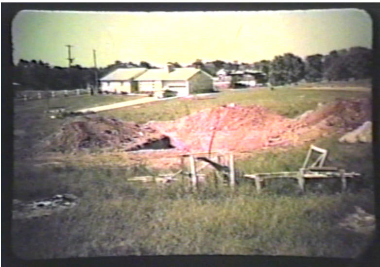
Construction in Matlock Heights, 1950s Courtesy of Carol and Richard Darling
