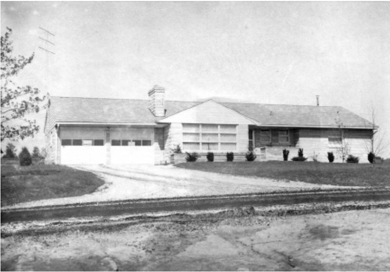
Limestone Facade, 2420 N Fritz Drive Bloomington HAND Department
