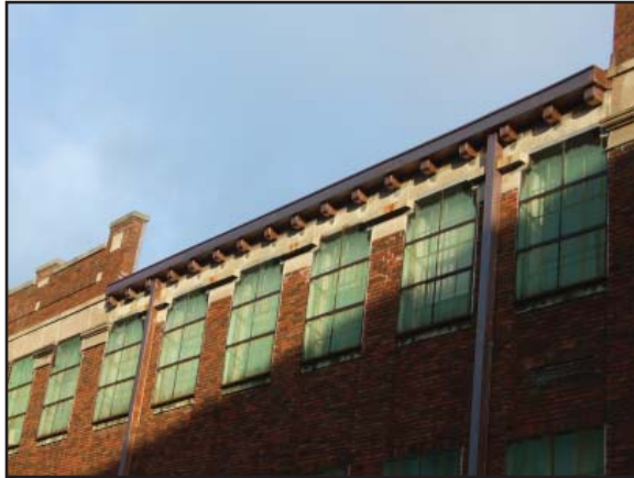
These storm windows obscure the design of the windows original to the building by utilizing divisions that conflict with the patterns of the original lights behind them.
