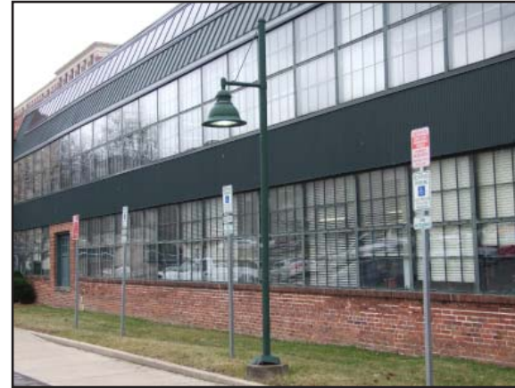
These new steel ventilator windows have exterior storms that provide additional insulation.
