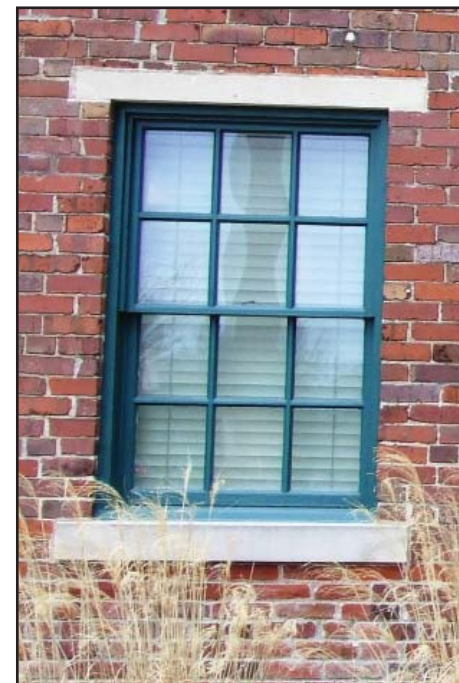
The double hung windows on Plant #1 are thermal pane, wood, true divided light windows that were approved through the tax credit process.
