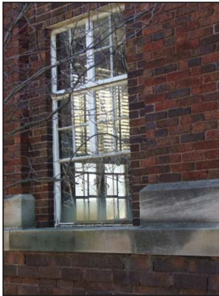
Windows on the front of the Administration Building are unusual double ventilator steel casements.
