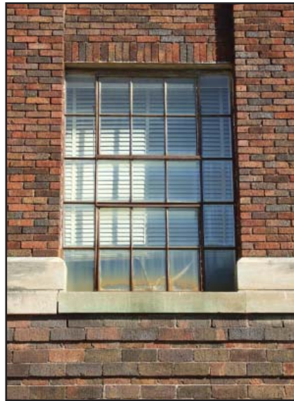
Some original sashes remain. They can be restored or provide templates for new windows.
