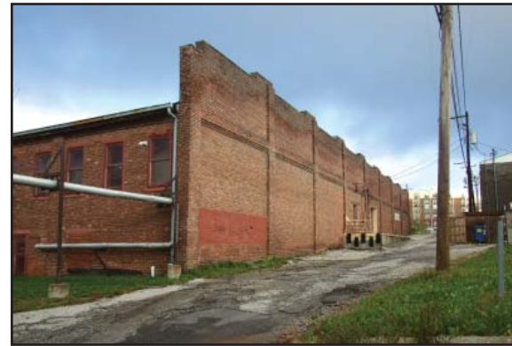
Exterior mechanicals, gutters and downspouts are original to the building and may be repaired or replaced, rather than hidden.
