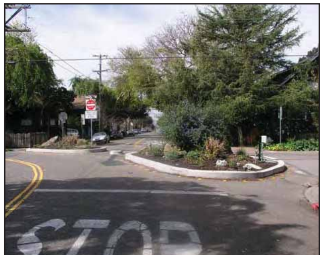
Bicycle Boulevard traffic diverters in Berkeley, CA
