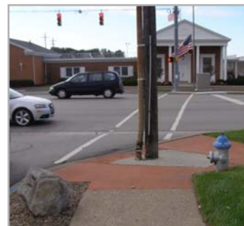
This curb ramp at 3rd & Pete Ellis was recently reconstructed, but the utility pole was not relocated.
