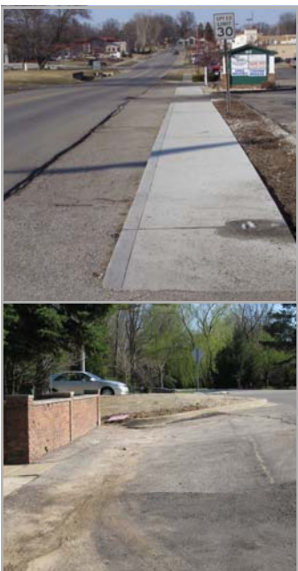
Incomplete sidewalk network along Woodscrest Dr.
