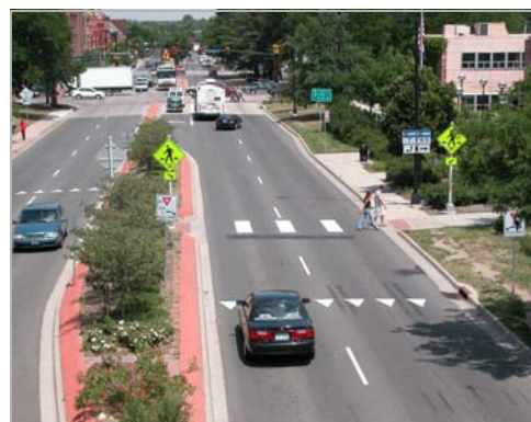
This crosswalk in Boulder, CO illustrates best practices for markings and signage at mid-block crosswalks.
