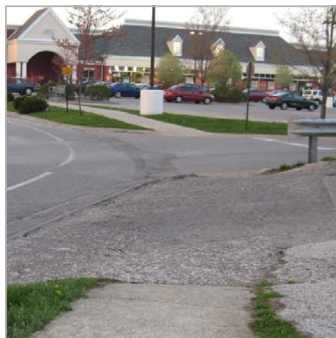
This series of driveway crossings along Kingston Dr. exhibits poor design. In particular, the sidewalk should continue through the crossings to indicate that the pedestrian has the right-of-way.
