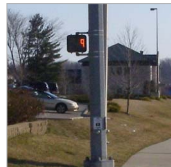
Pedestrian signals with countdown timers, as here at 2nd St. & College Mall Rd., provide valuable information for pedestrians and motorists .
