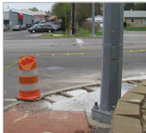
Curb ramp reconstruction at 3rd St. & Clarizz Blvd.
