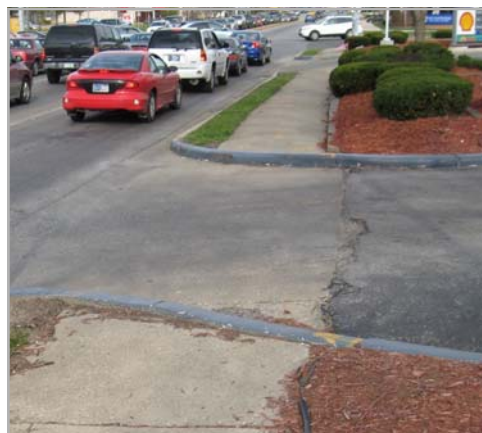
Curb ramps are needed at this driveway crossing along E. 3 rd St.
