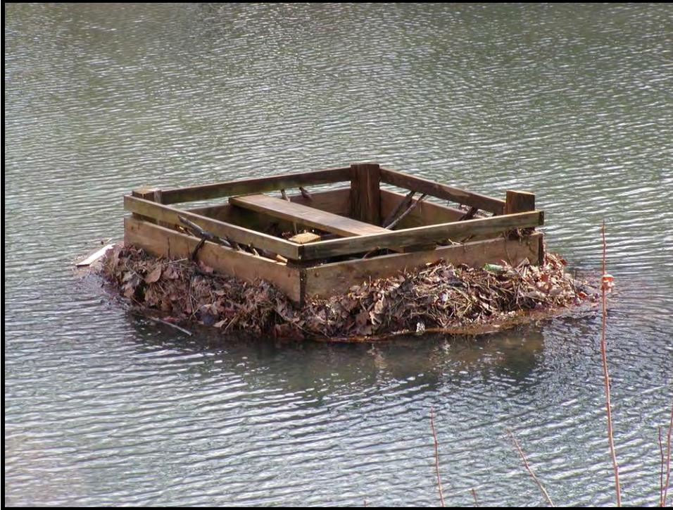
**Figure 22. Clogged water control structure in the Tamarron retention basin.**
