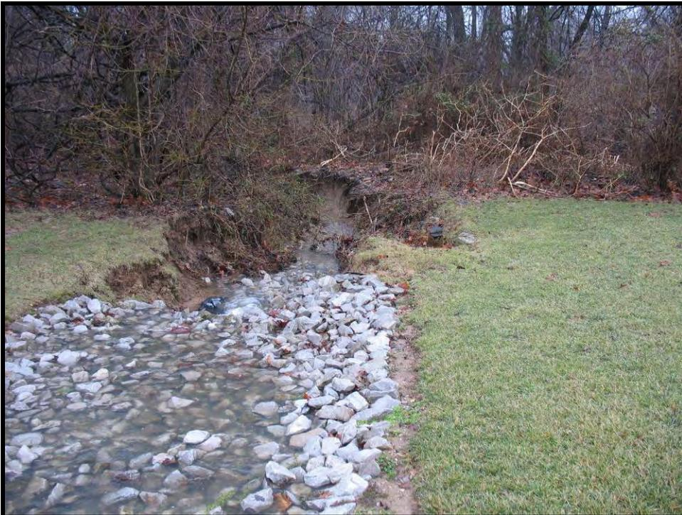
**Figure 14. Runoff from the Indiana University (IU) Foundation drains via a rip-rap lined ditch but substantial erosion is apparent where the rip-rap ends.**
