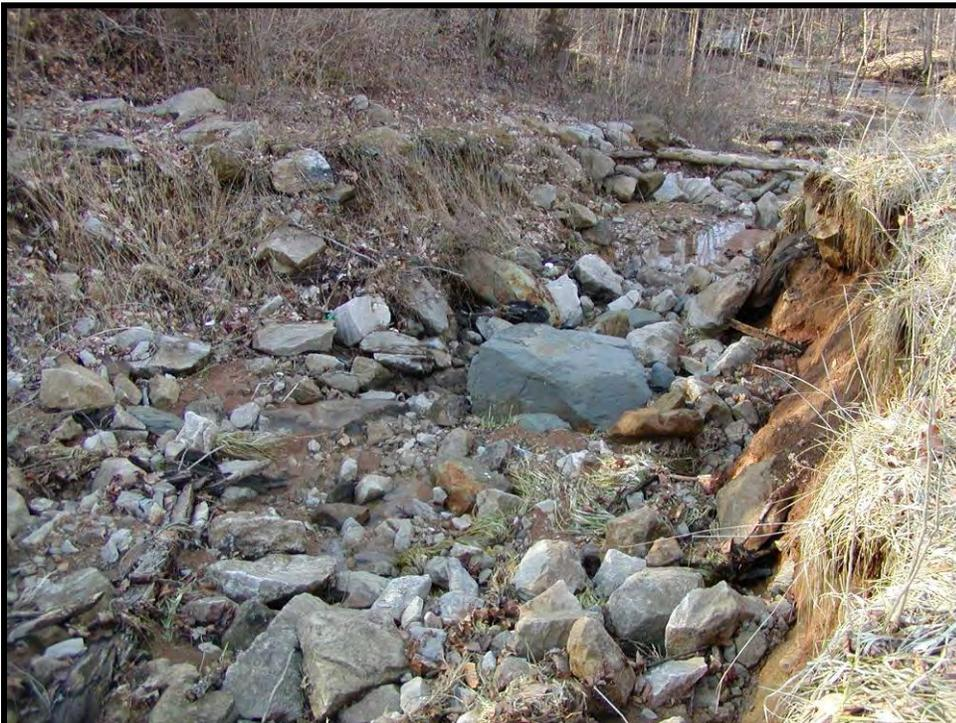
**Figure 23. Eroded Tamarron retention pond outlet.**
