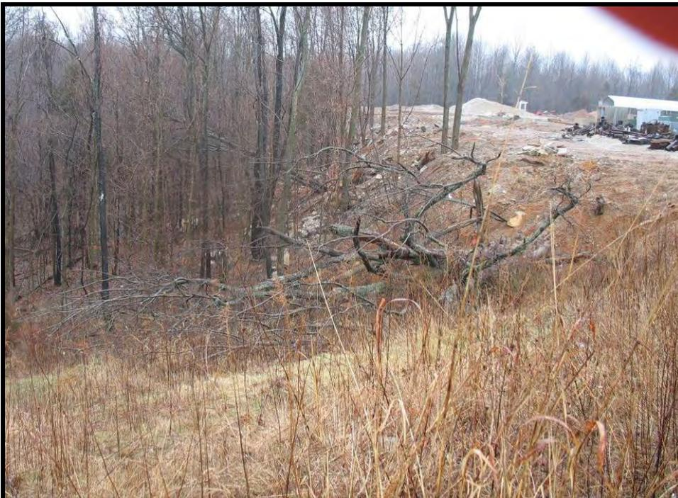
**Figure 17. Equipment storage area leveled with fill dirt left a steep, unprotected embankment that erodes into Griffy Creek.**
