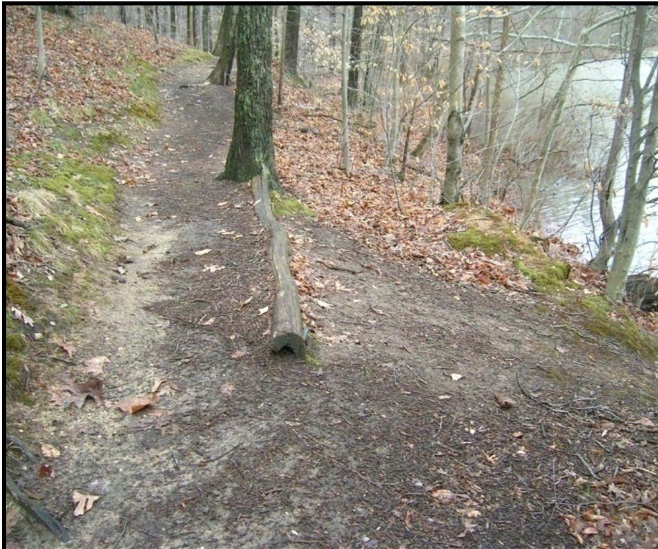
**Figure 81. Logs installed to maintain downhill edge of trail.**
