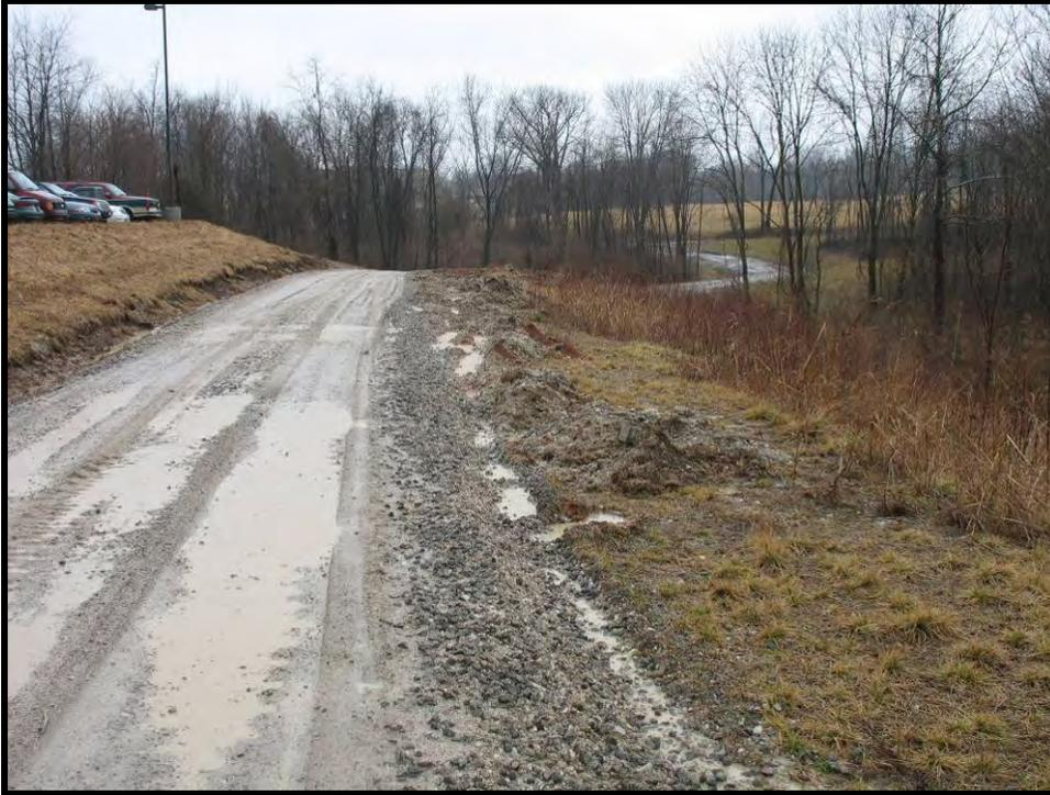
**Figure 16. A gravel road to the storage area at the new IU Physical Plant building is unstable and erodes into Griffy Creek.**
