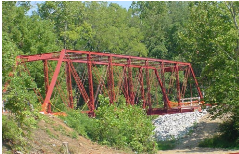
Example of a Gateway Bridge on Clear Creek Trail.
