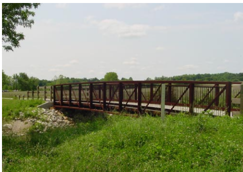
Example of a Standard Bridge on Clear Creek Trail.
