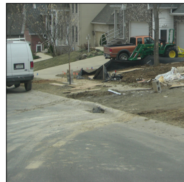
Builders are required to install appropriate erosion control measures.
