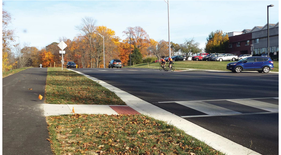
Improvements for all transportation modes at 17th Street and Jordan Avenue. A new sidewalk was installed on the north side of 17th Street, and the new crosswalks help make crossing the street safer and easier for pedestrians at this busy intersection.
