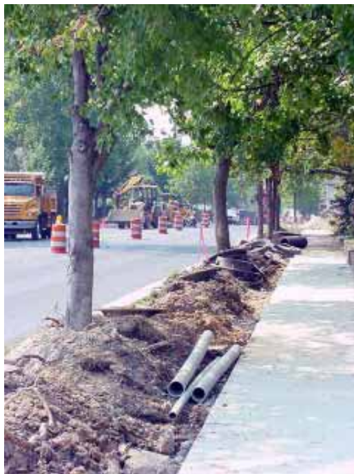
W. Kirkwood Ave. streetscape project
