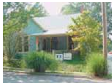
A HAND structure rehabilitation project in Prospect Hill
