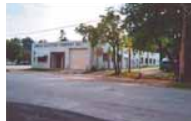
Former Owens Electric Building
