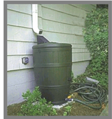
Source: U.S. EPA. A rain barrel used to collect rooftop runoff using a gutter/downspout system.
