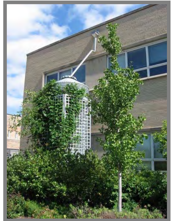
Commercially sized cistern at the Chicago Center for Green Technology. Source: Abby Hall, EPA.
