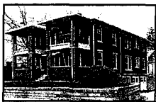
1. The Angelika Apartments 111 East Tenth ca. 1928
