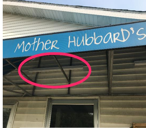
New lighting above the office door
