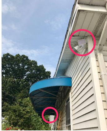
New motion lighting on south side of building
