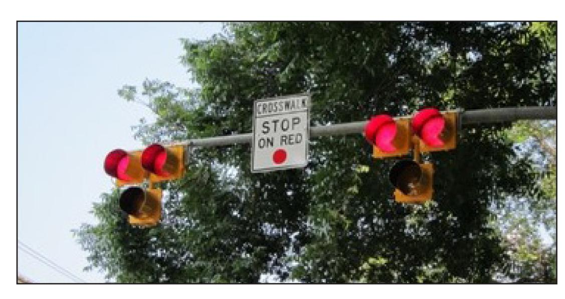
The pedestrian hybrid beacon (a.k.a. the High intensity Activated crossWalK (or HAWK) is a pedestrian-activated warning device located on the roadside or on mast arms over midblock pedestrian crossings.
