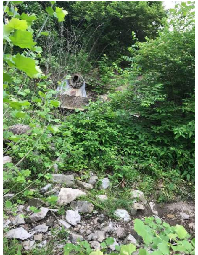
Photopoint 22: Taken facing east, north of E Moores. Steep incline up to road. Photo taken 5/21/2018. B-25
