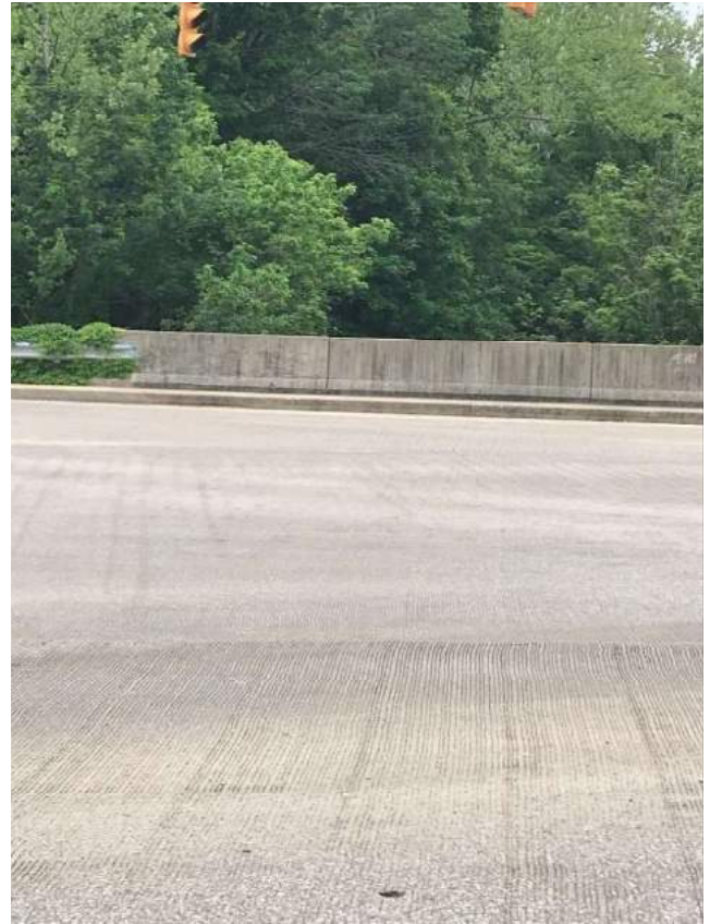
Photopoint 24: Taken facing south, north of E Moores Pike towards E Moores Pike overpass.
