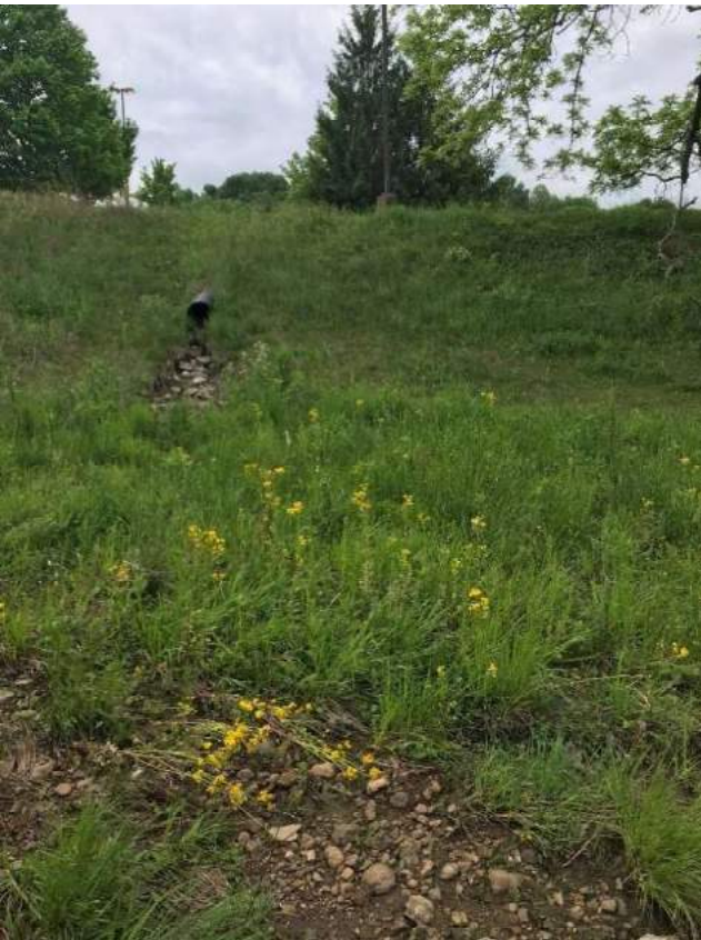
Photopoint 9: Taken north of UNT1 facing south across UNT1. Flow coming from culvert does not reach UNT1 as a defined channel. Photo taken 5/21/2018.
