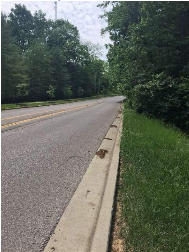
Photopoint 68: Taken facing south on Sare Rd. No roadside ditches present. Photo taken 5/21/2018.
