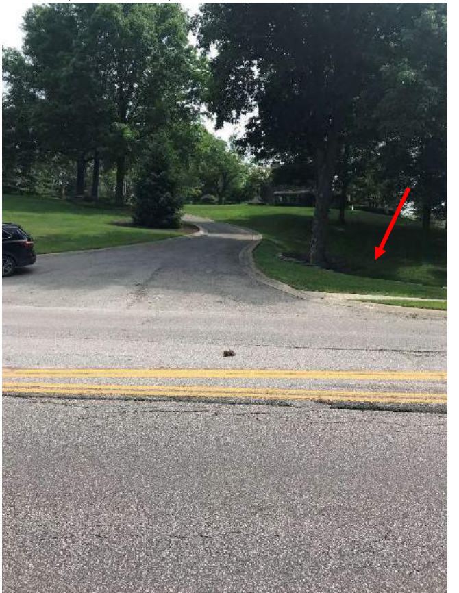
Photopoint 69: Taken facing east on Sare Rd. Red arrow points to UNT4 culvert. Photo taken 5/21/2018. B-37
