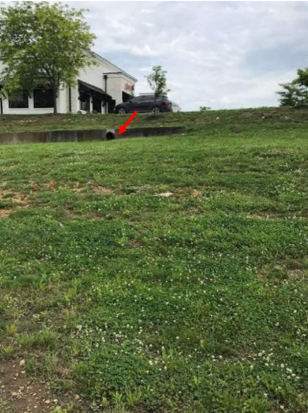
Photopoint 7: Taken north of UNT1 facing north. No apparent channel from culvert (red arrow). Photo taken 5/21/2018.
