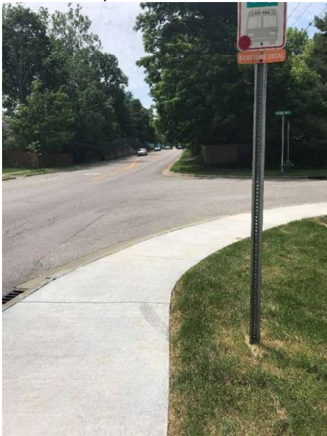
Photopoint 60: Taken facing south on Sare Rd looking past Spicewood Lane. No roadside ditches present. Photo taken 5/21/2018.
