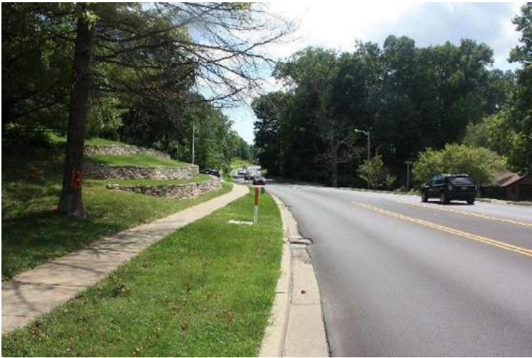
Photopoint 72: Taken facing south on Sare Rd. No roadside ditches present. Photo taken 8/30/2018.
