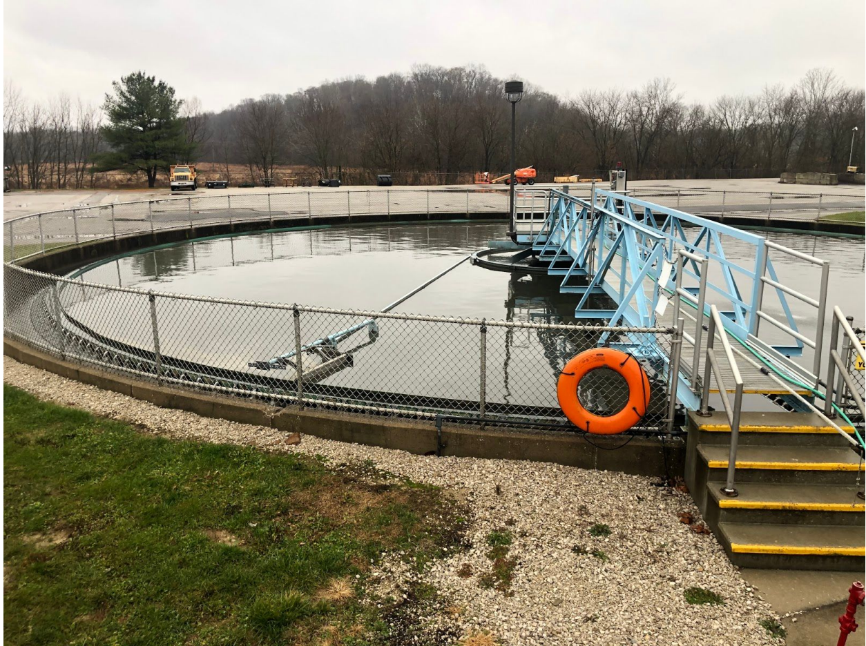
Figure 5. A primary clarifier at the Blucher Poole WWTW.
