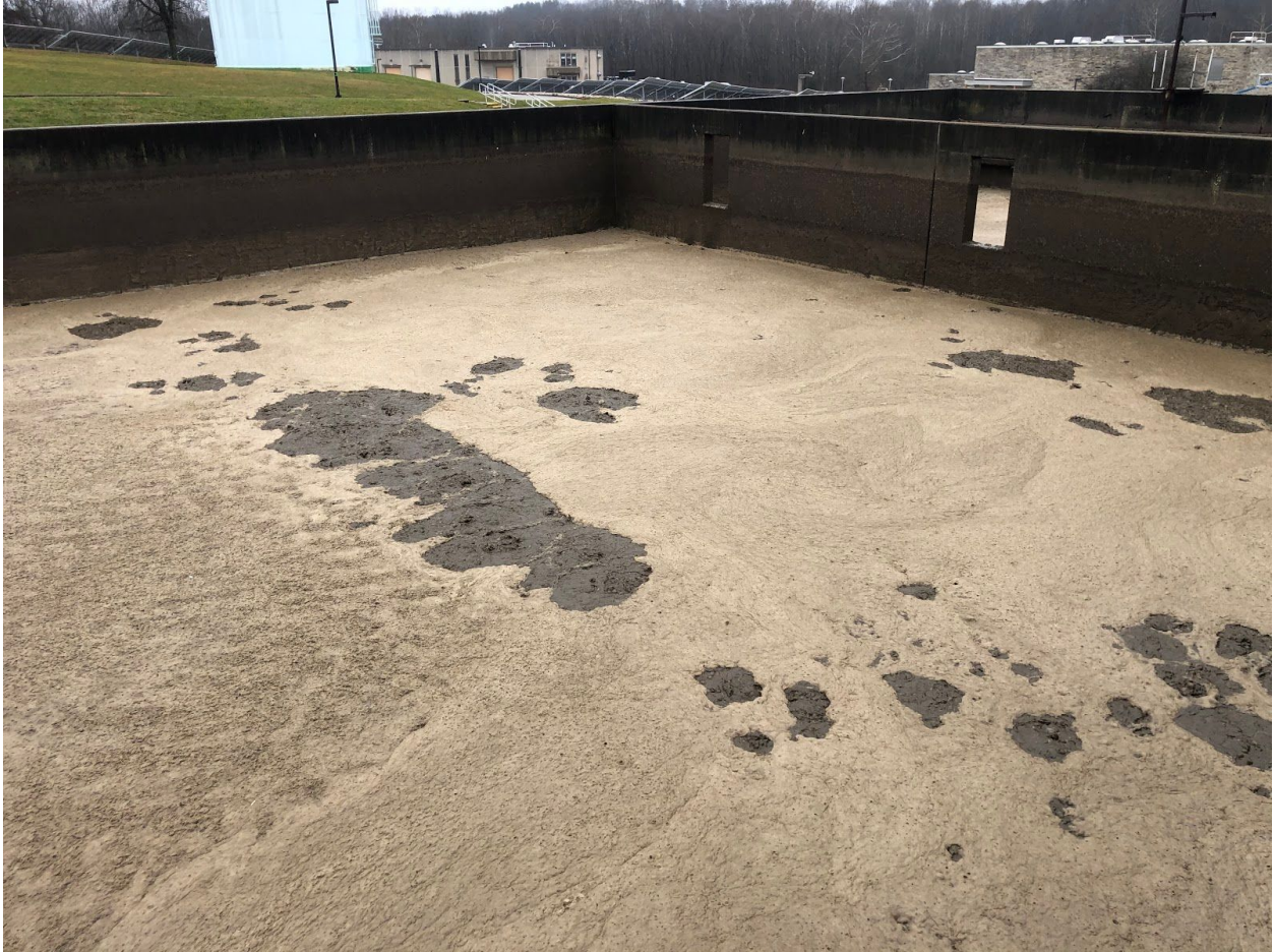
Figure 9. Aerobic digestion of wasted sludge at Dillman Road WWTP.
