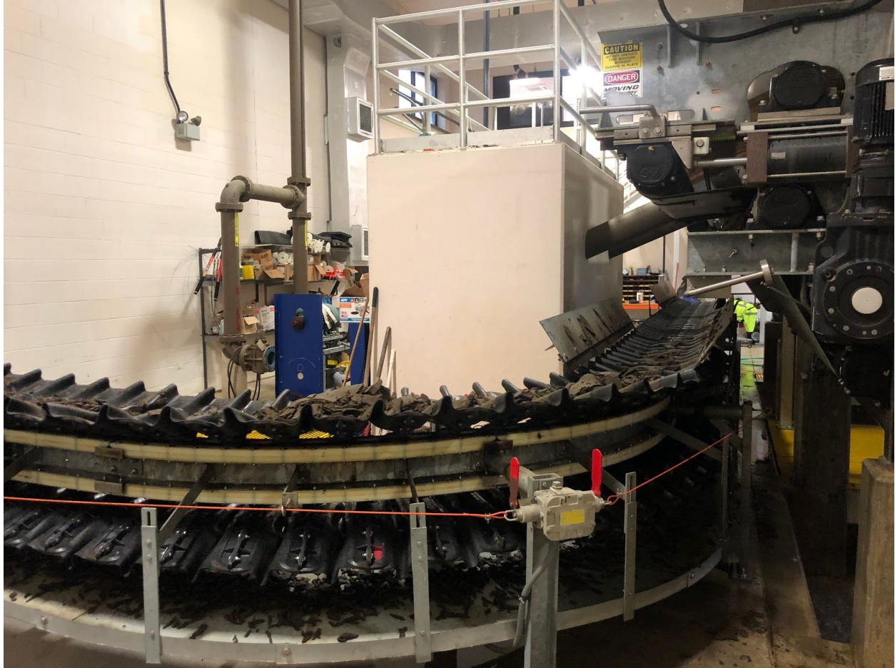
Figure 10. Waste sludge leaving the belt press at Dillman Road WWTP.
