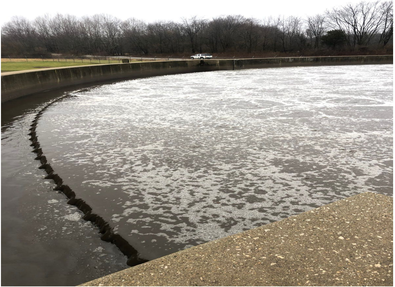
Figure 6. Aeration and overflow of activated sludge at the Blucher Poole WWTP.
