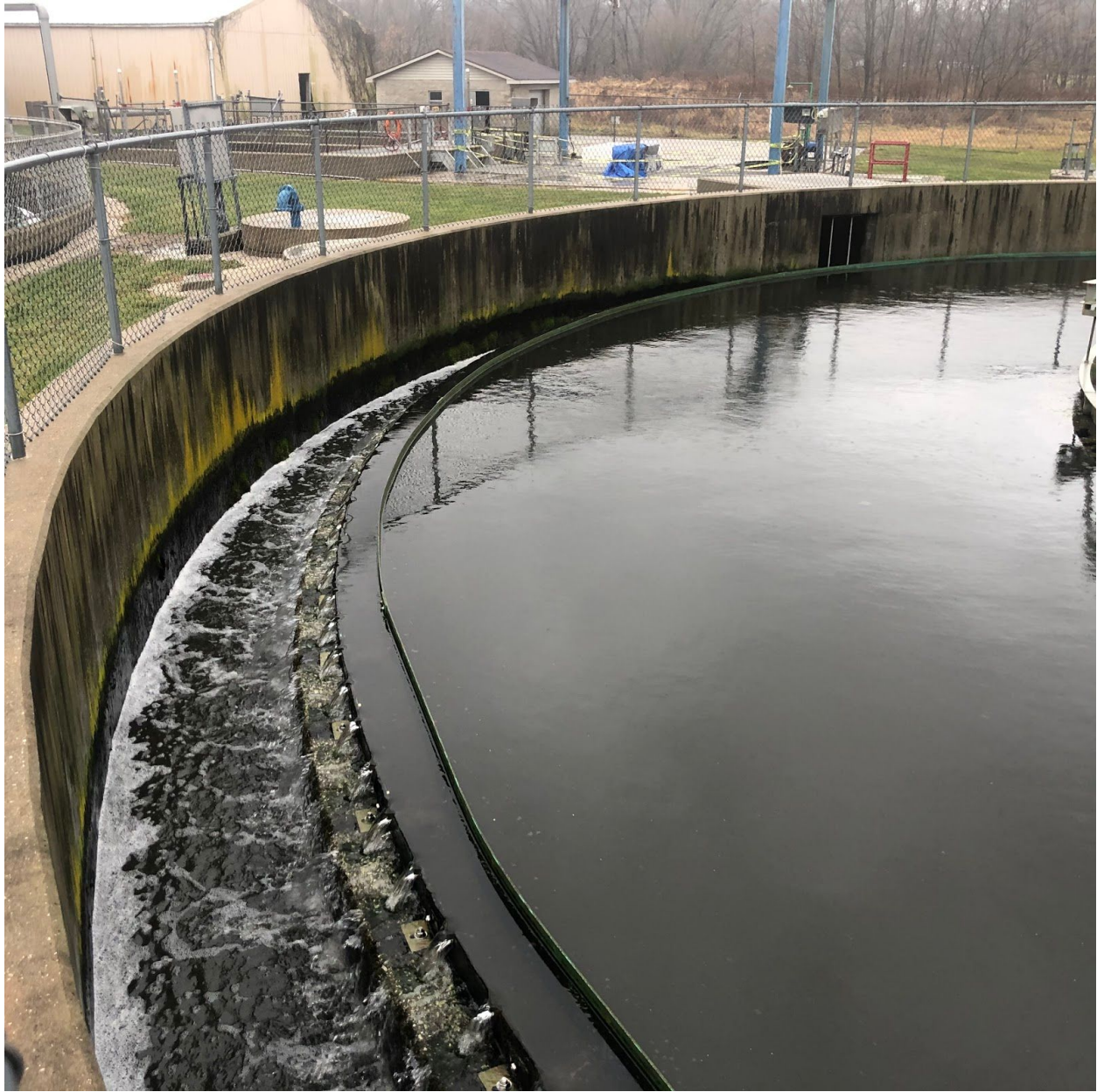
Figure 7. Treated effluent exiting the secondary clarifier at the Blucher Poole WWTP.
