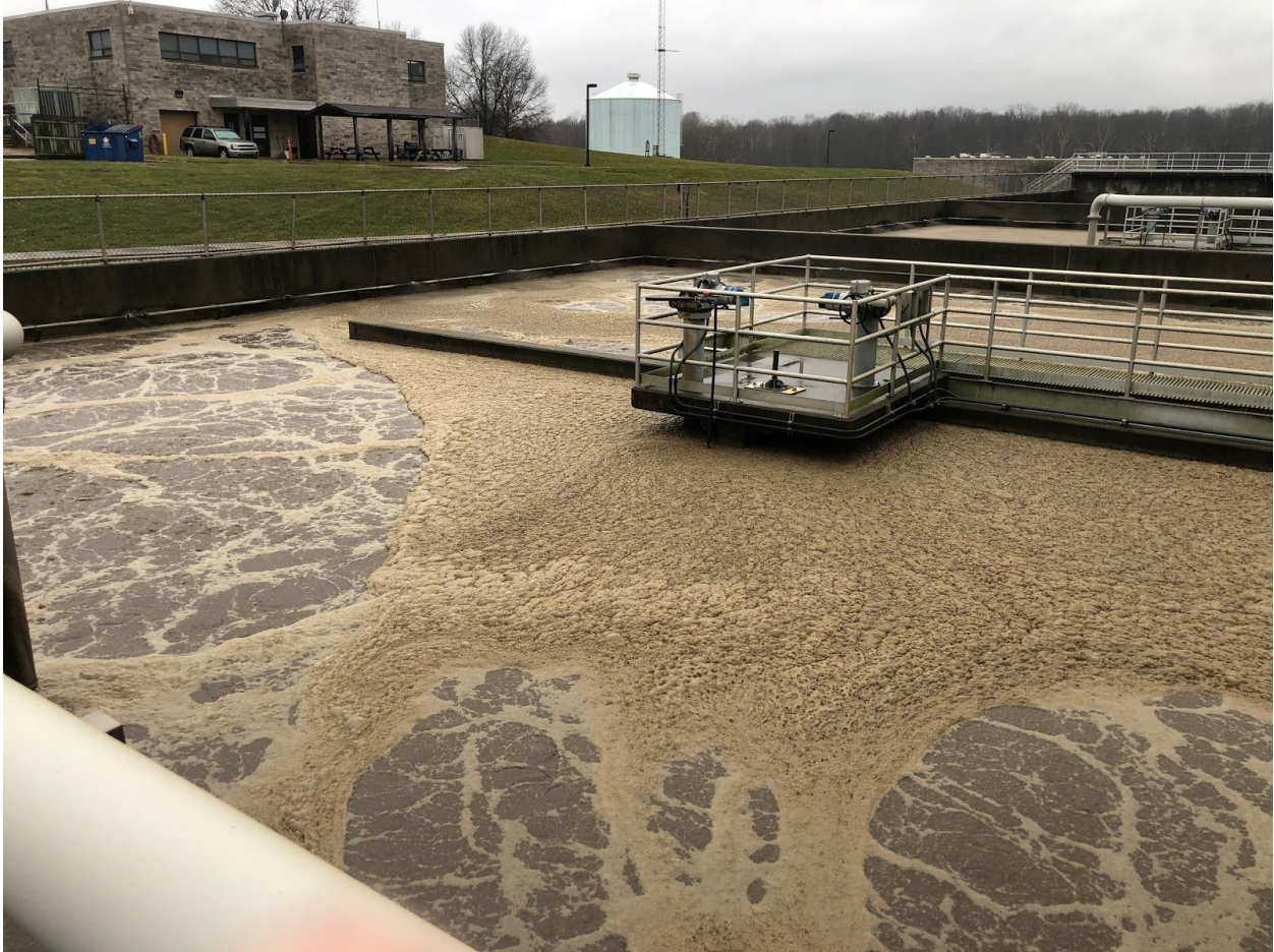
Figure 8. Aeration of activated sludge at the Dillman Road WWTP.
