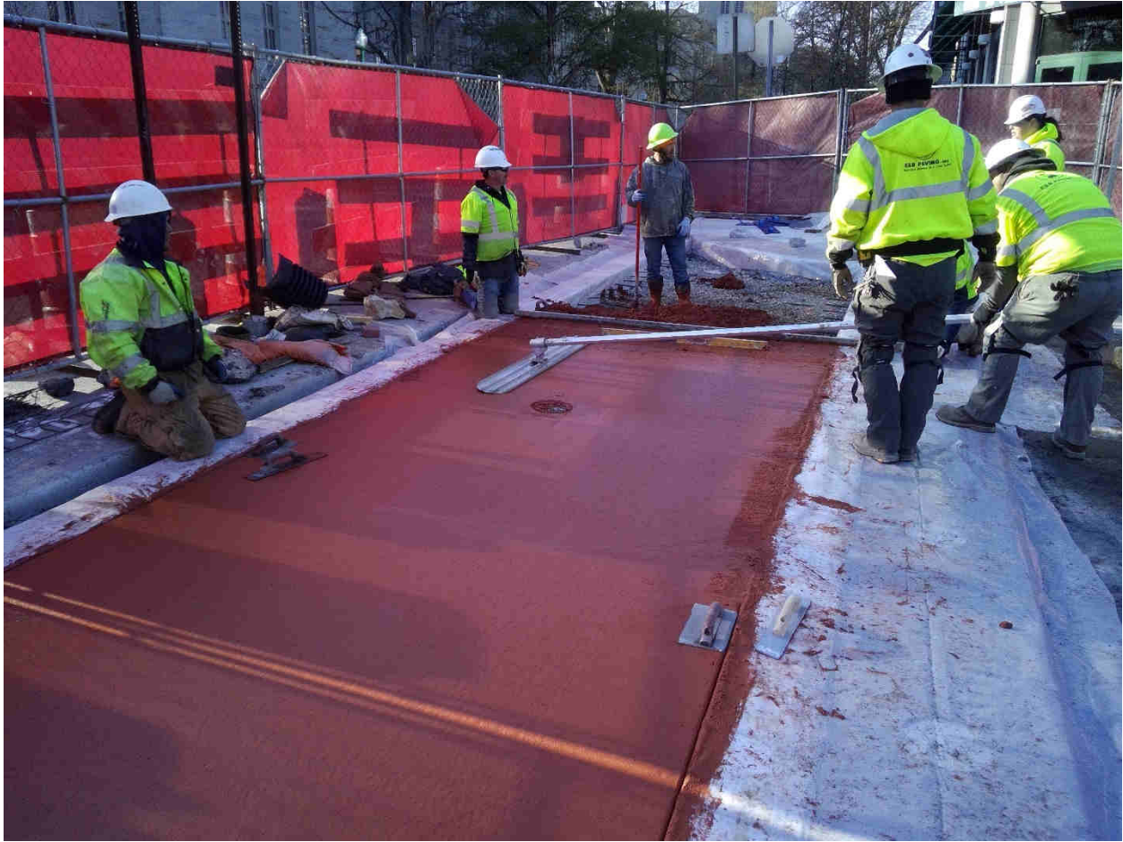
Indiana Avenue crosswalk under construction.
