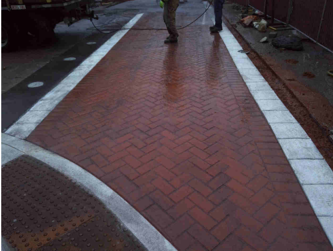
Indiana Avenue, curb ramps, bollard footer and crosswalk; finished.
