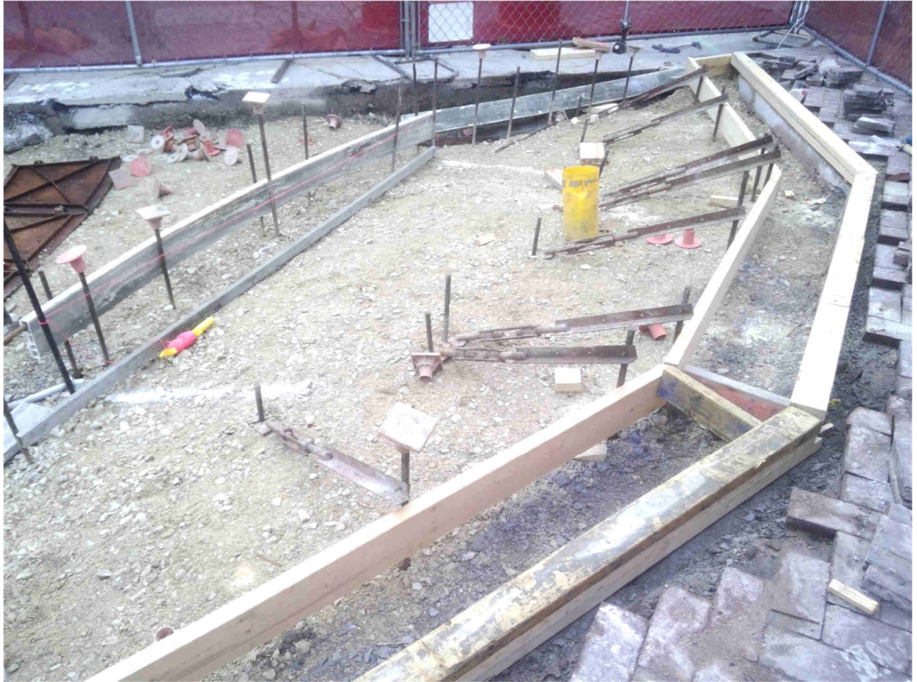
Indiana Avenue, South curb ramp under construction.
