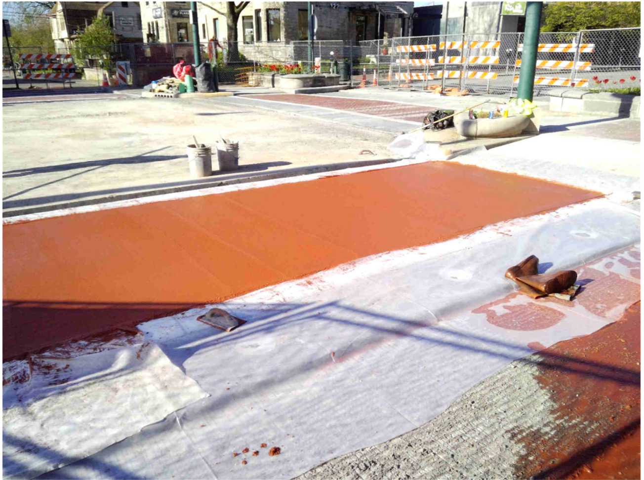
Crosswalk at North leg Grant St. Intersection under construction.
