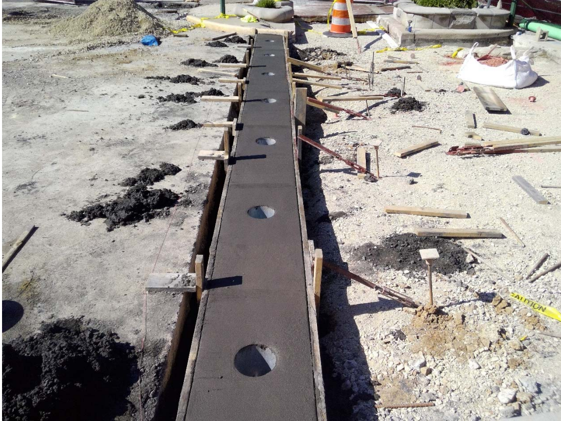
Bollard footer recently constructed at Dunn St., Intersection, East leg.
