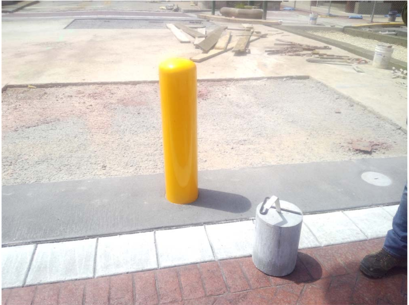
An example of how a bollard change is accomplished.
