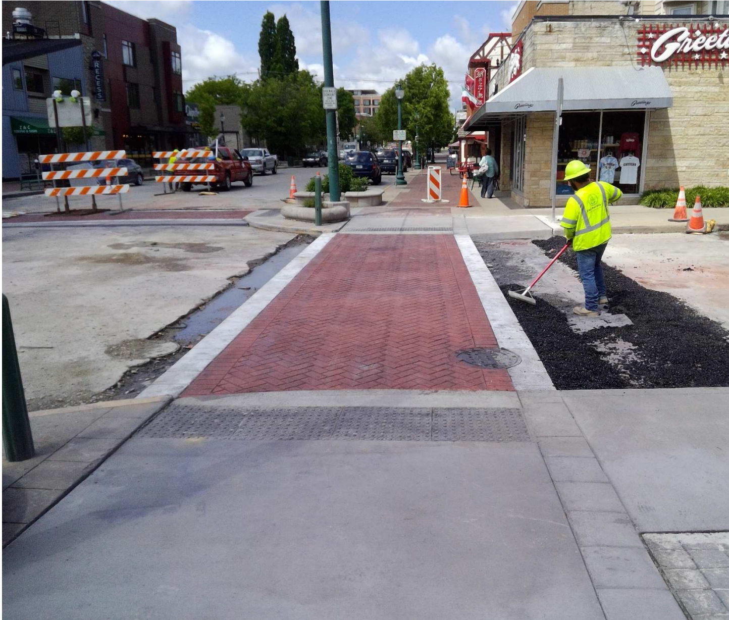
North leg, Dunn St. Intersection, under construction.
