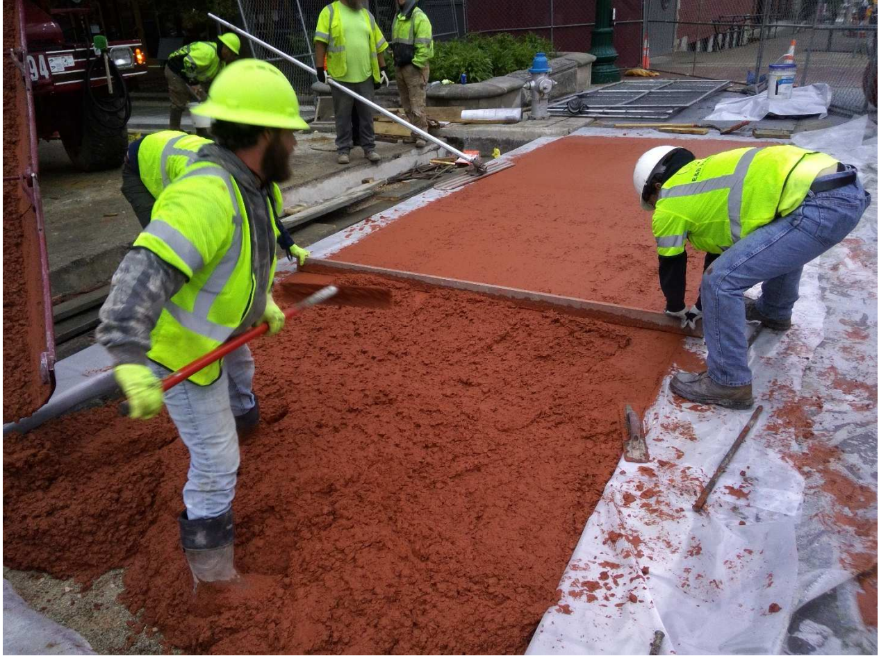
Crosswalk under construction at Walnut, East leg.
