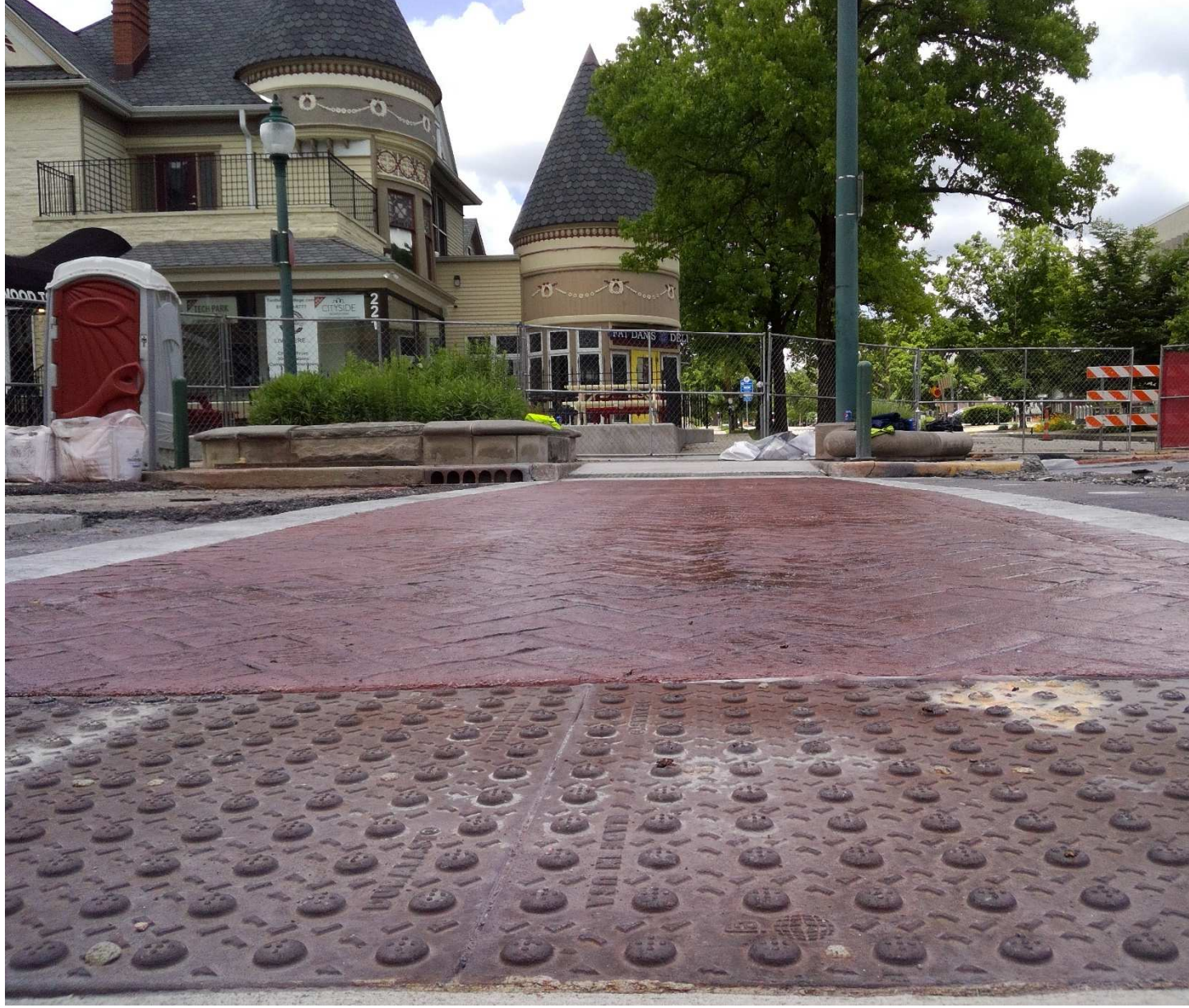
West leg, Lincoln, crosswalk and curb ramps sealed and finished.
