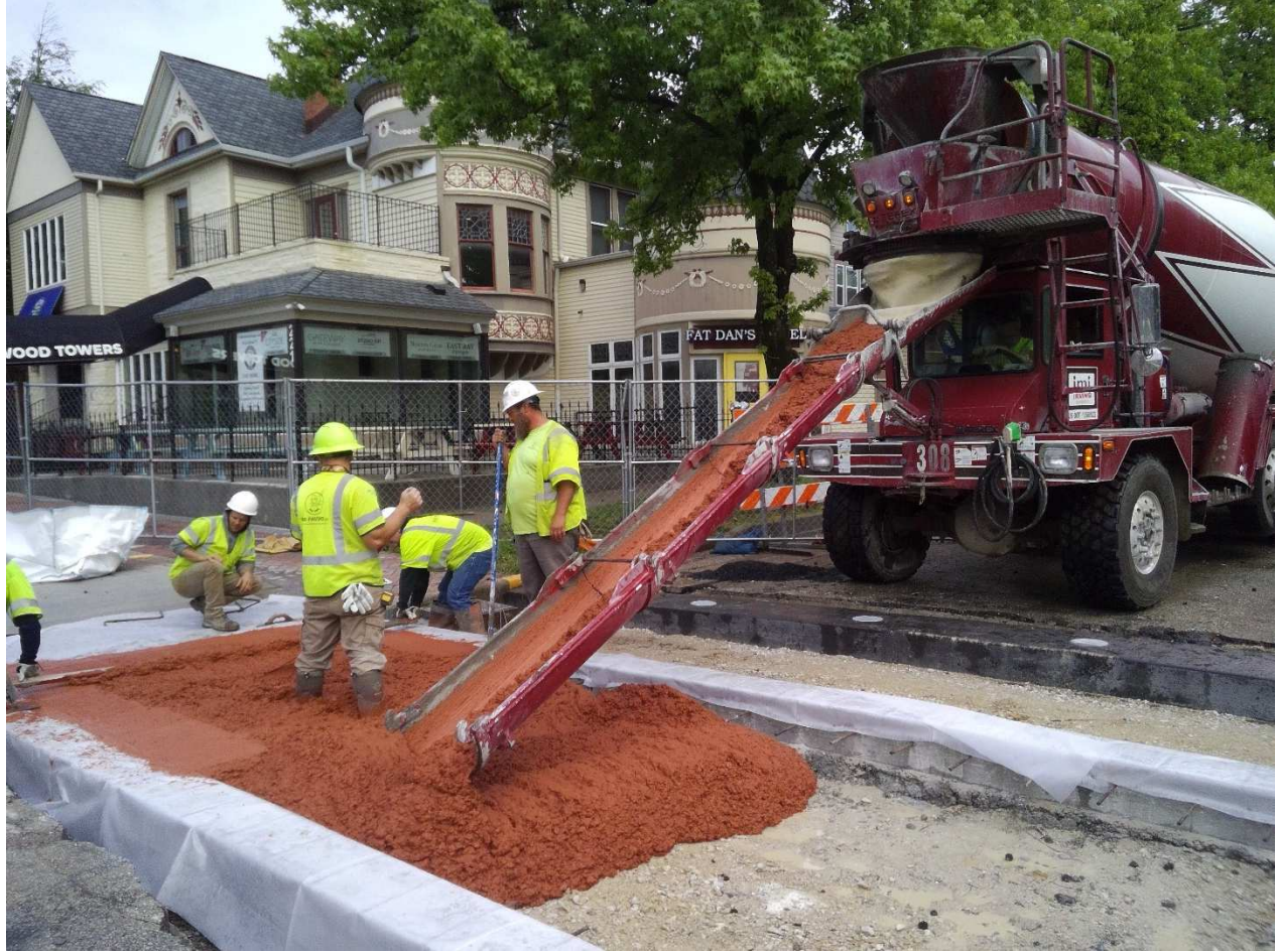
The last crosswalk going in at North leg, Lincoln Ave.
