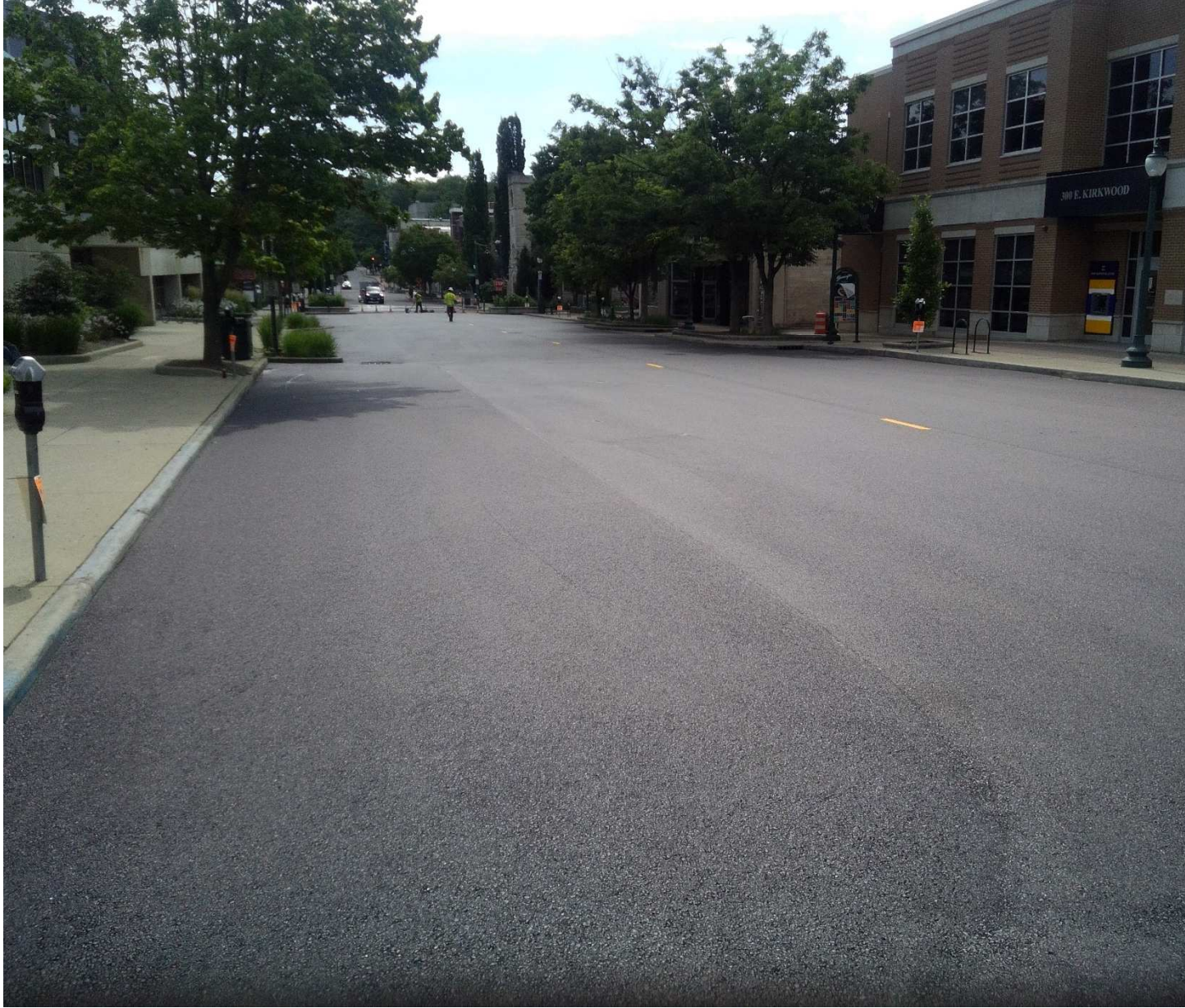
HMA surface 9.5mm laid.
