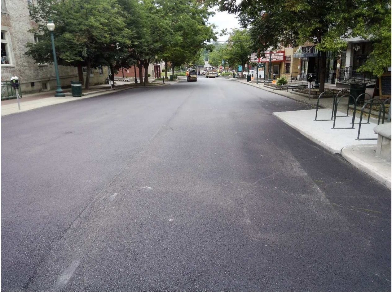
HMA Surface, 9.5mm Mainline, laid at the West end of Kirkwood.
