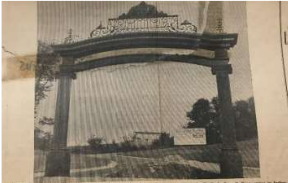
BEAUTIFUL IRON GATES adorn the entrance to the newly opened first addition of the Blue Ridge Estates on the north side of Bloomington off of Highway 37. Construction of the entrance is now completed and work on 72 lots on over 300 acres of
