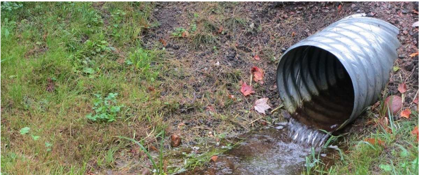
An Example of an Installed Driveway Culvert
