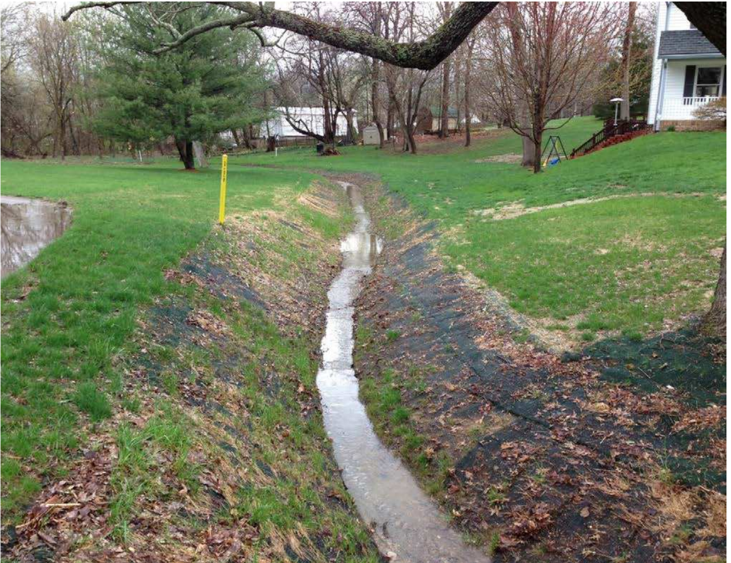
An example of ditch stabilization in progress
