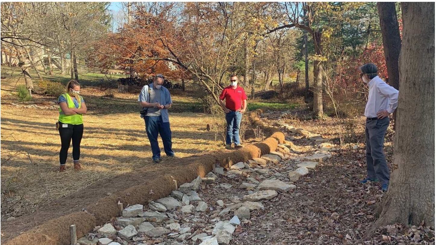
A Dry Creek Bed in Progress
