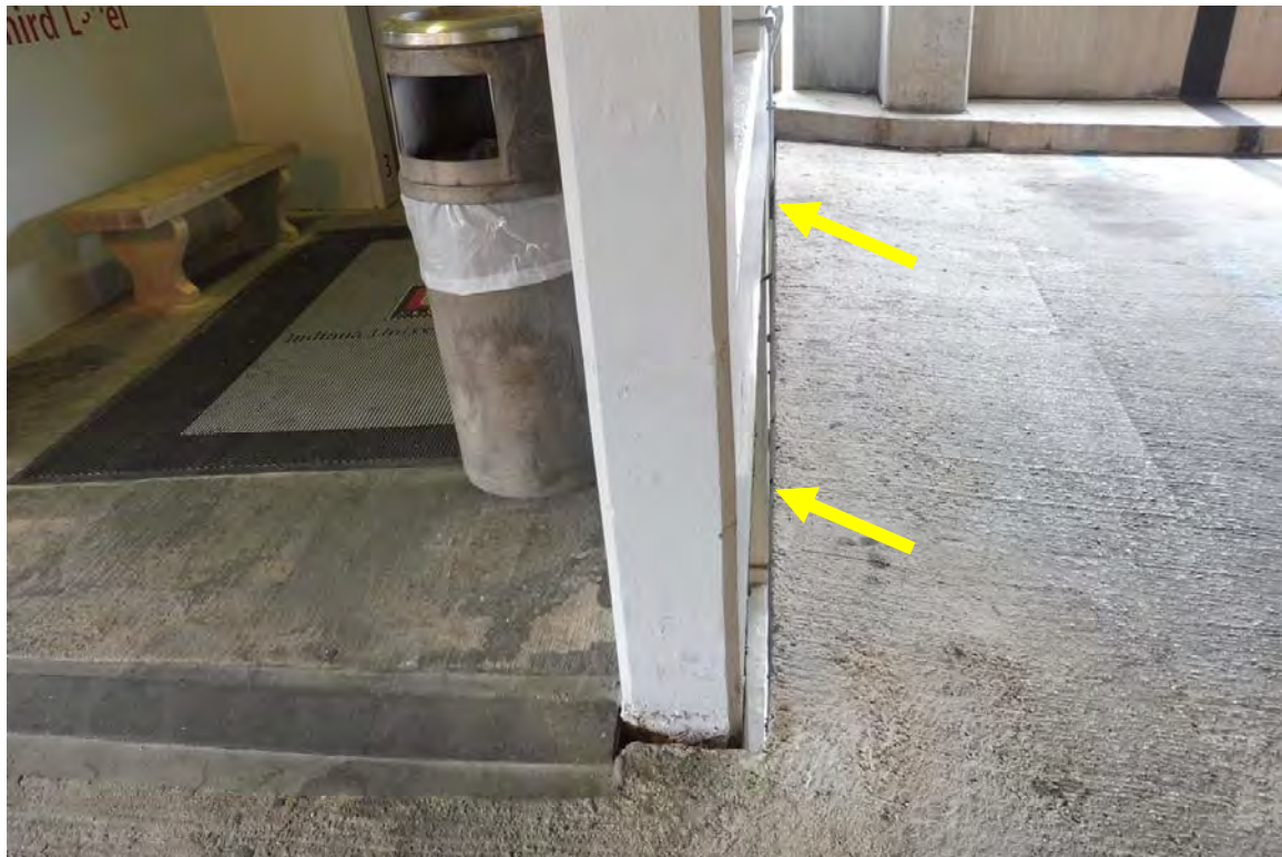
Photo 110 The expansion joint between the southwest stair/elevator tower and the garage floor slab is open at Levels 2 and 3. We would suggest an expansion joint be installed to seal the gap.
