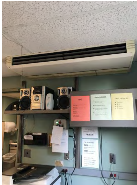
Indoor fan-coil for heat pump
