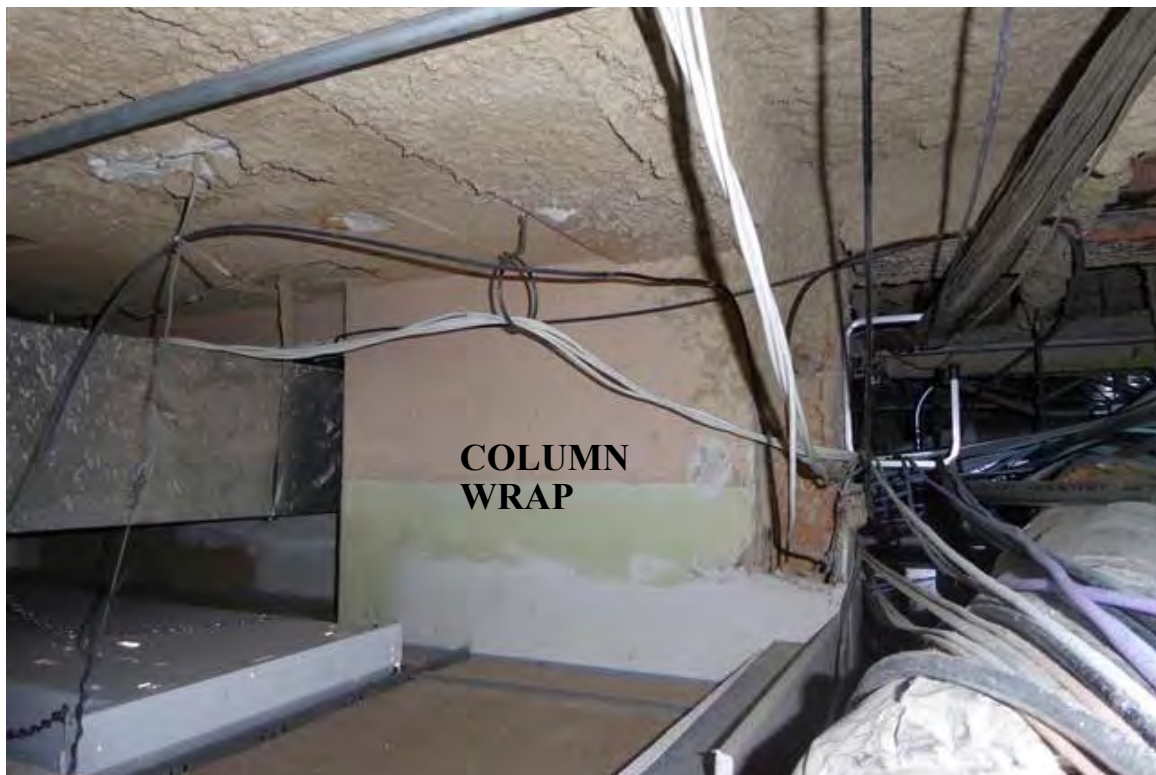
Photo 54 Steel framing supports the second floor, third floor and roof levels. The steel columns are wrapped with clay tile and plaster for fire protection.
