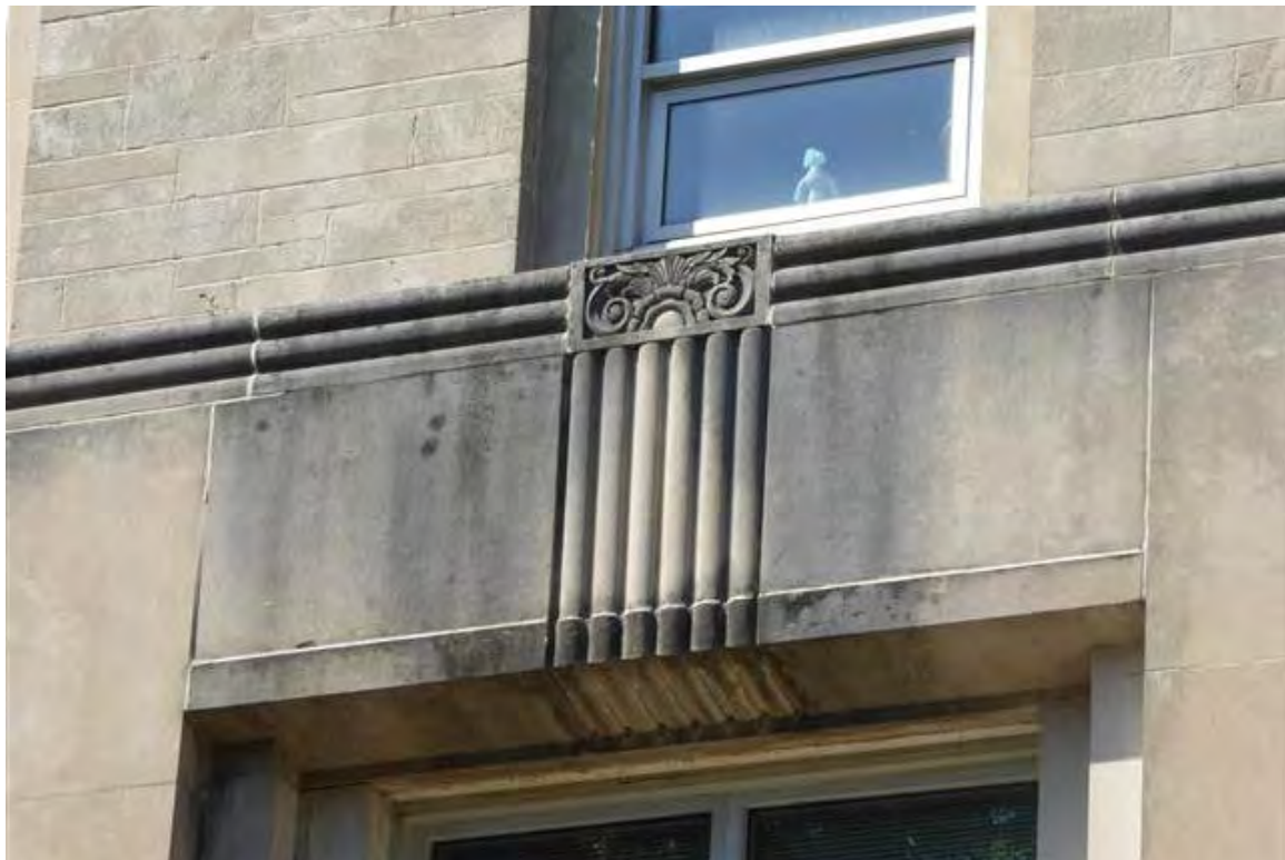
Photo 32 Organic material grows on the face of the protrusion over the east entrance.
