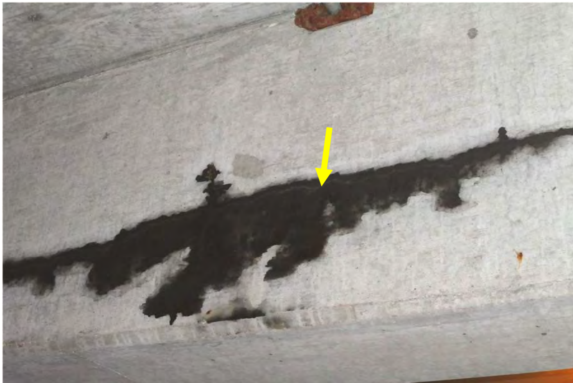
Photo 66 Close-up view of Photo 7. Note the crack seen through the grease staining.
