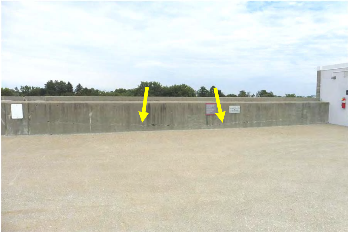
Photo 63 Post-tensioned beam along the north elevation at the roof deck has a crack that appears to follow the drape of the post-tensioning tendons. Grease is leaching from the crack near midspan, meaning that the sheathing has failed possibly due to moisture entering the unbonded tendons.
