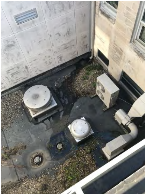
Heat pump, on right
