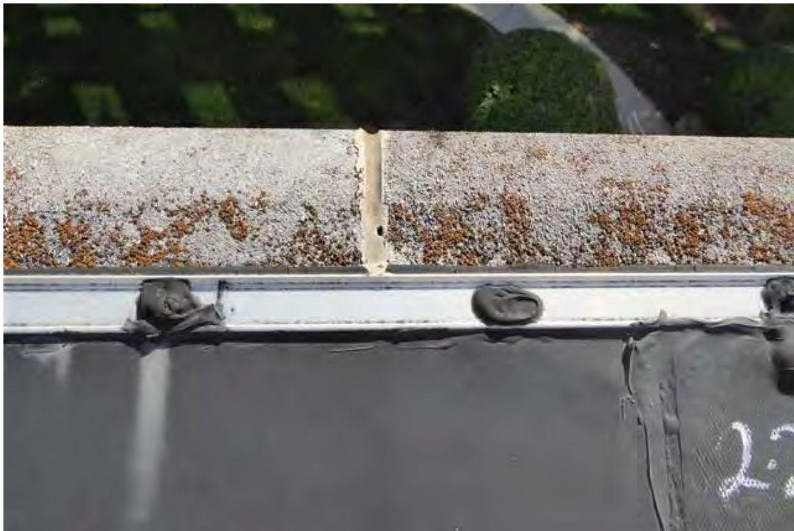
Photo 14 The membrane turns up over the back and top of the limestone coping and is secured with a termination bar.
