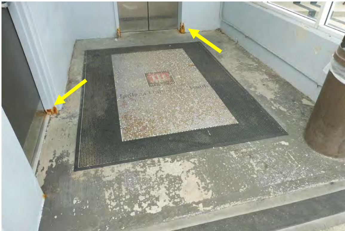
Photo 100 The existing floor coating throughout the stair/elevator tower has failed. Corrosion of the door frames both to the stair and the elevator were observed on each level.
