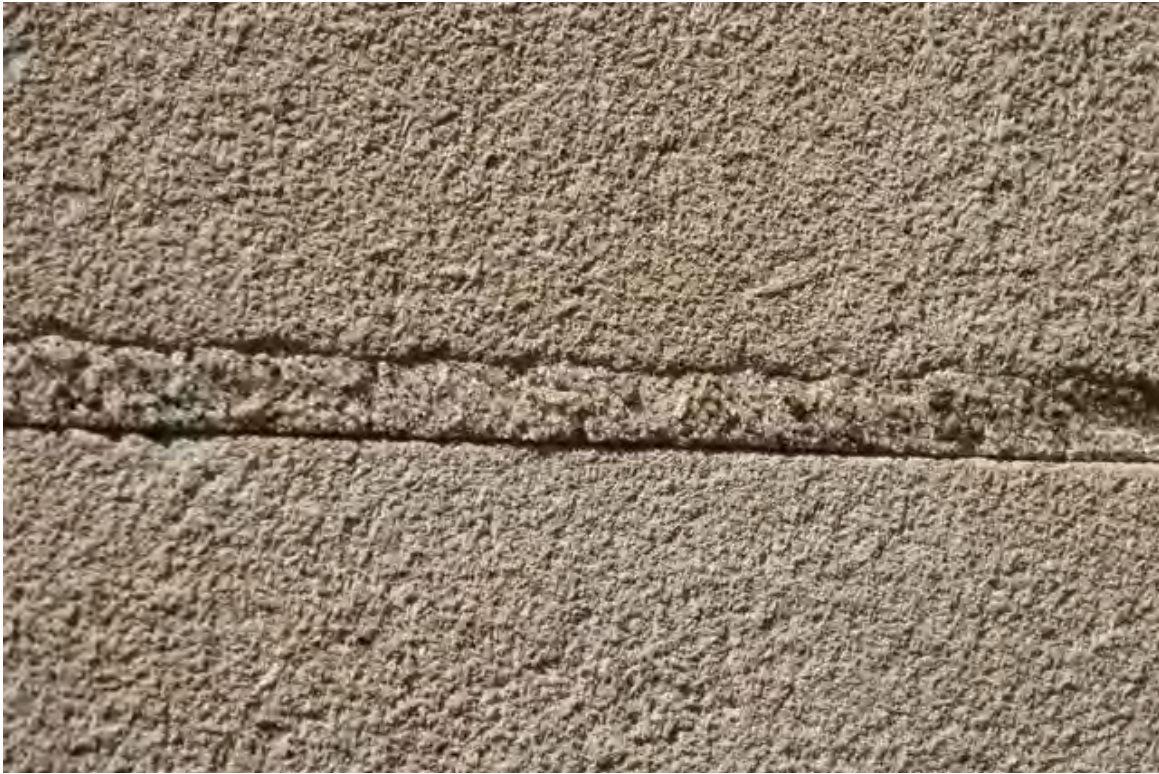
Photo 25 A few of the joints were struck flush and are more prone to moisture infiltration.
