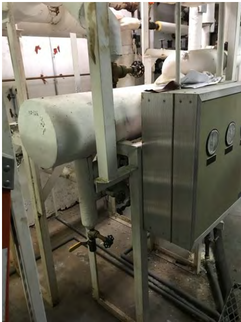
Steam-to-Hot Water Heat exchanger
