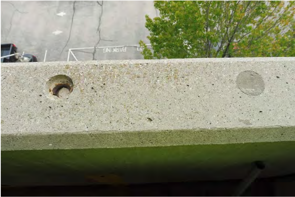
Photo 87 Missing grout pockets at the lift insert holes on the skyward face of the façade panels...
