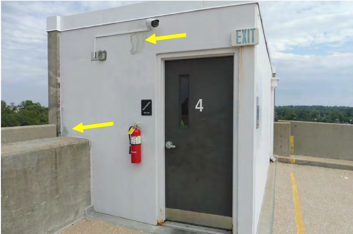
Photo 111 Northeast stair tower at the roof level. The coating on the concrete walls has failed in multiple areas on the outside of the stair tower.
