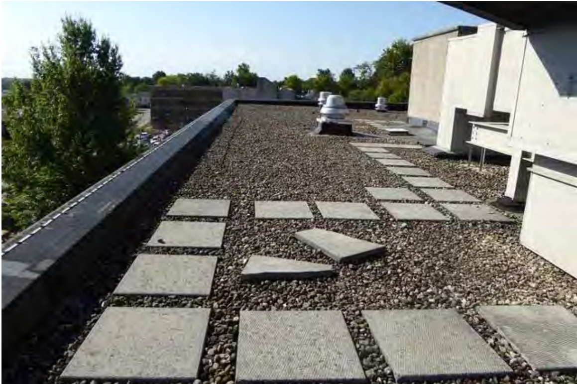
Photo 13 The roof is covered with a ballasted EPDM. The roof is reported to be at least 30 years old.
