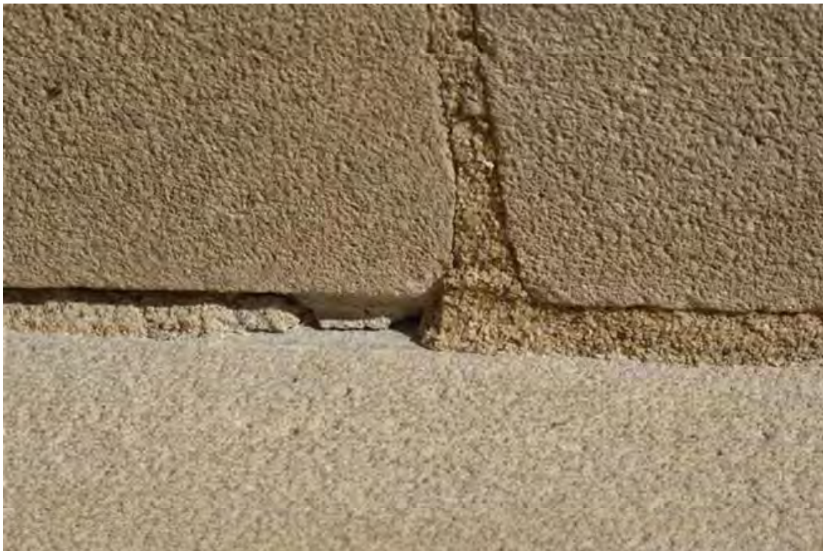
Photo 26 More recent tuckpointing has been thin and tends to crack and fall back out of the joint.
