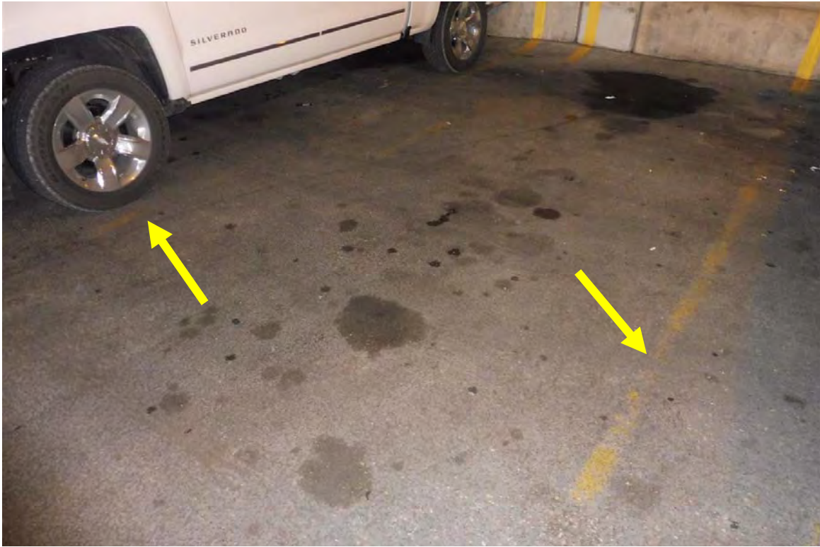
Photo 81 The striping paint throughout the garage should be reinstalled as many of the parking stall lines have faded/worn away.
