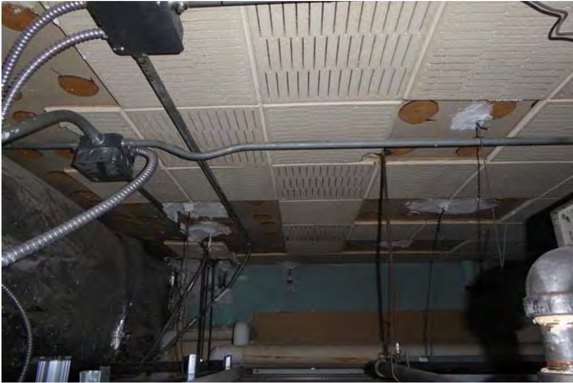
Photo 53 Typical view above the drop ceiling. The original glue on ceiling tile and plaster ceilings are still in place.
