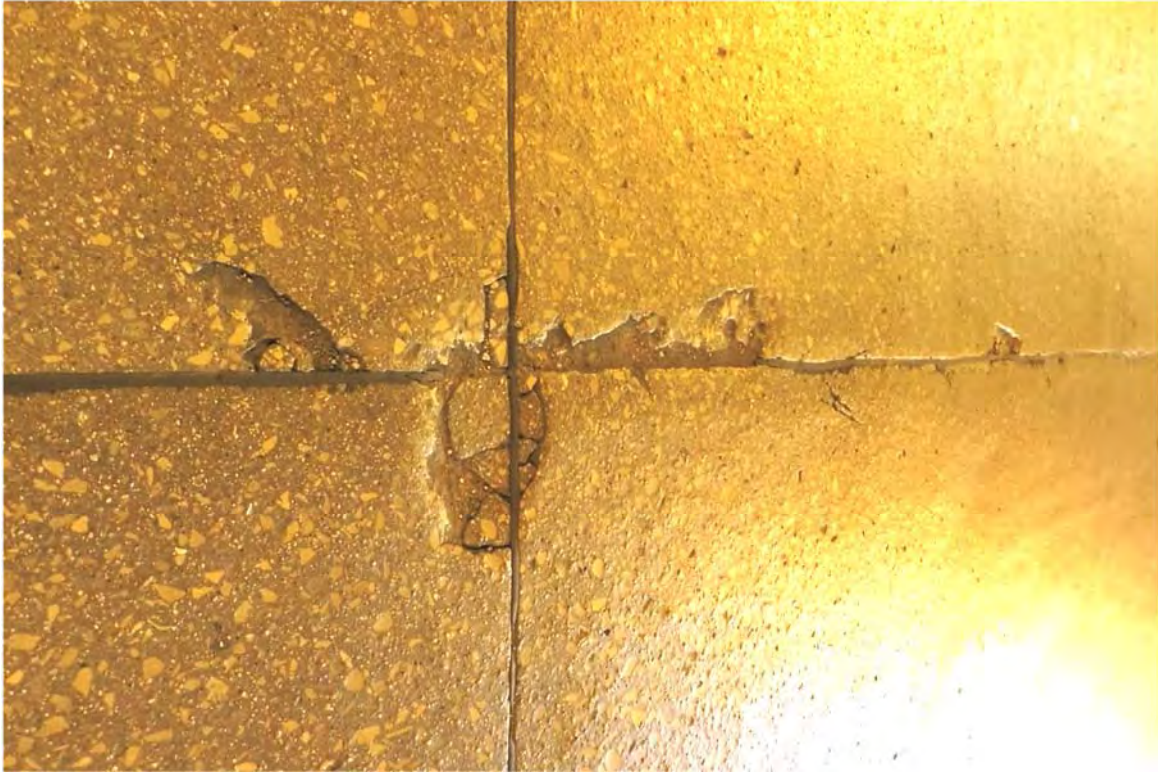
Photo 77 Small spalls in the slab-on-grade at the sawcut control joints should be patched to keep from enlarging with time.
