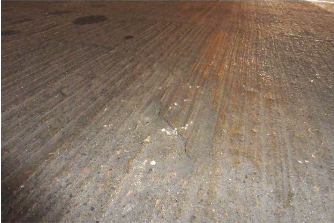
Photo 75 Slab scaling of the top surface was noted at some locations, generally on the lower levels where the volume of vehicles is typically higher.
