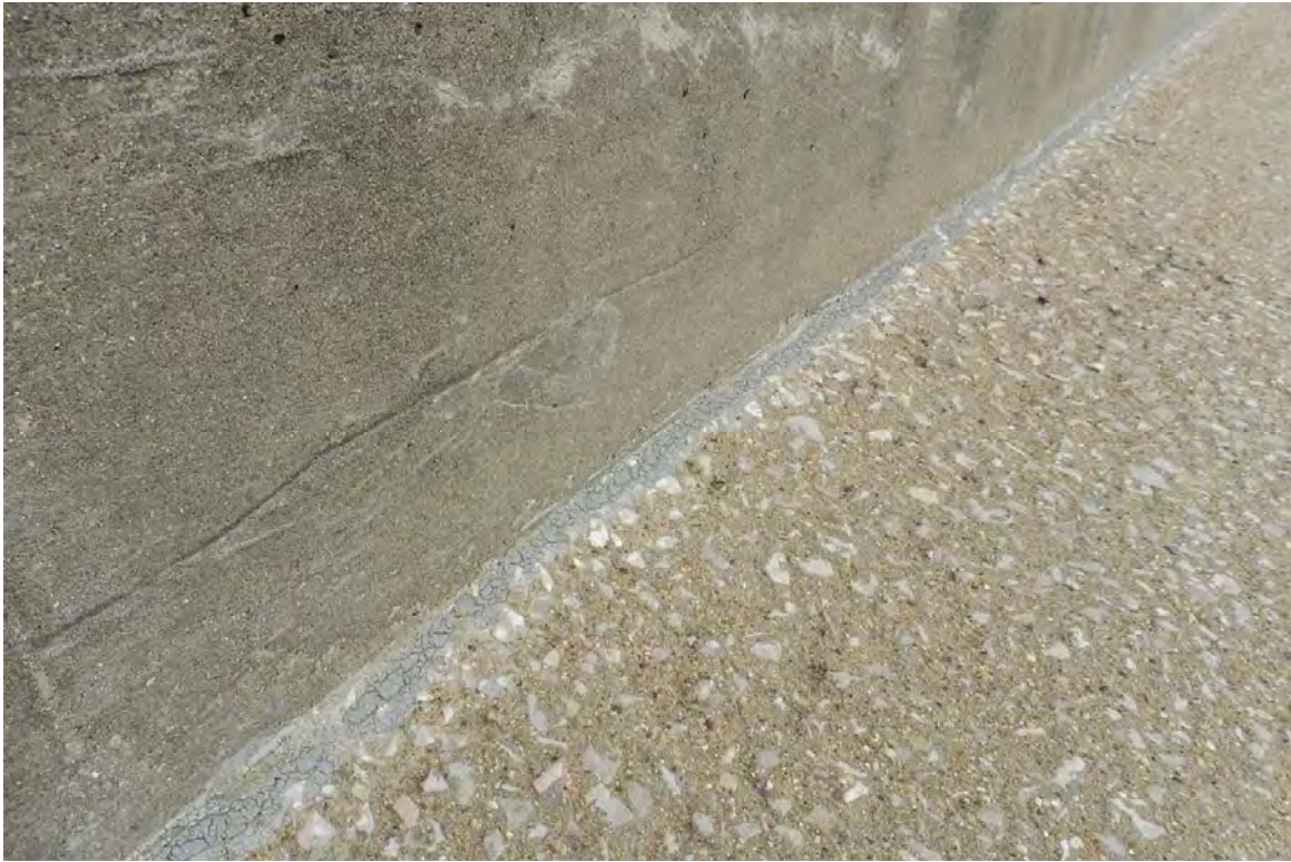
Photo 71 The perimeter sealant joints, however, are in fair to poor condition as many have failed such as the joint seen here on the roof level.
