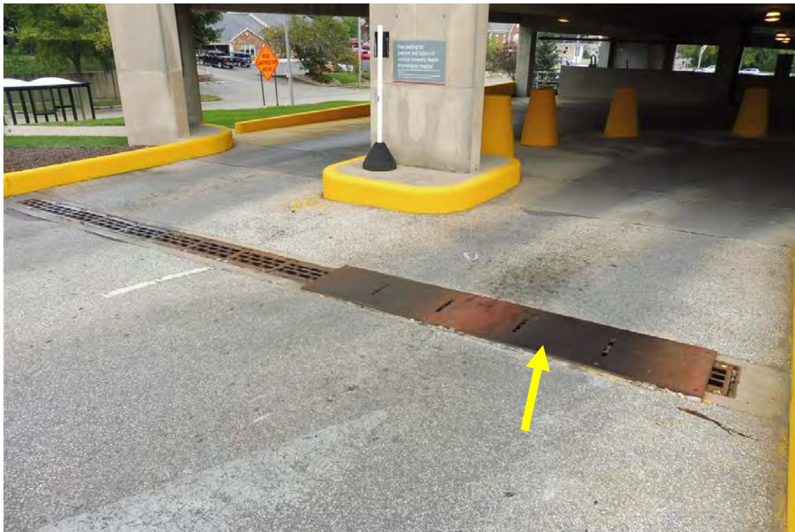
Photo 78 Steel road plate installed over the trench drain at the main entrance. The plate was loose and needs to be re-anchored. The condition of the trench drain below the road plate was not visible.
