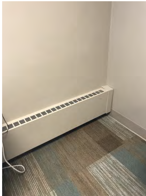
Perimeter hot water heater
