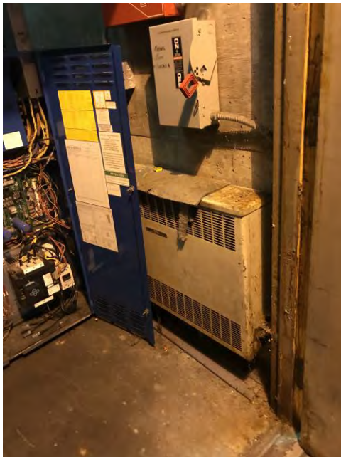
Elevator machine room heater
