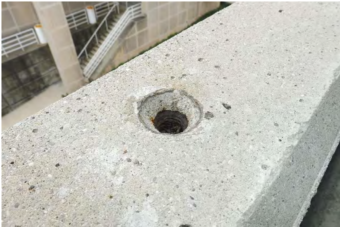
Photo 88 ...should be cleaned and filled with non-shrink grout to keep the metal insert embedment from corroding.
