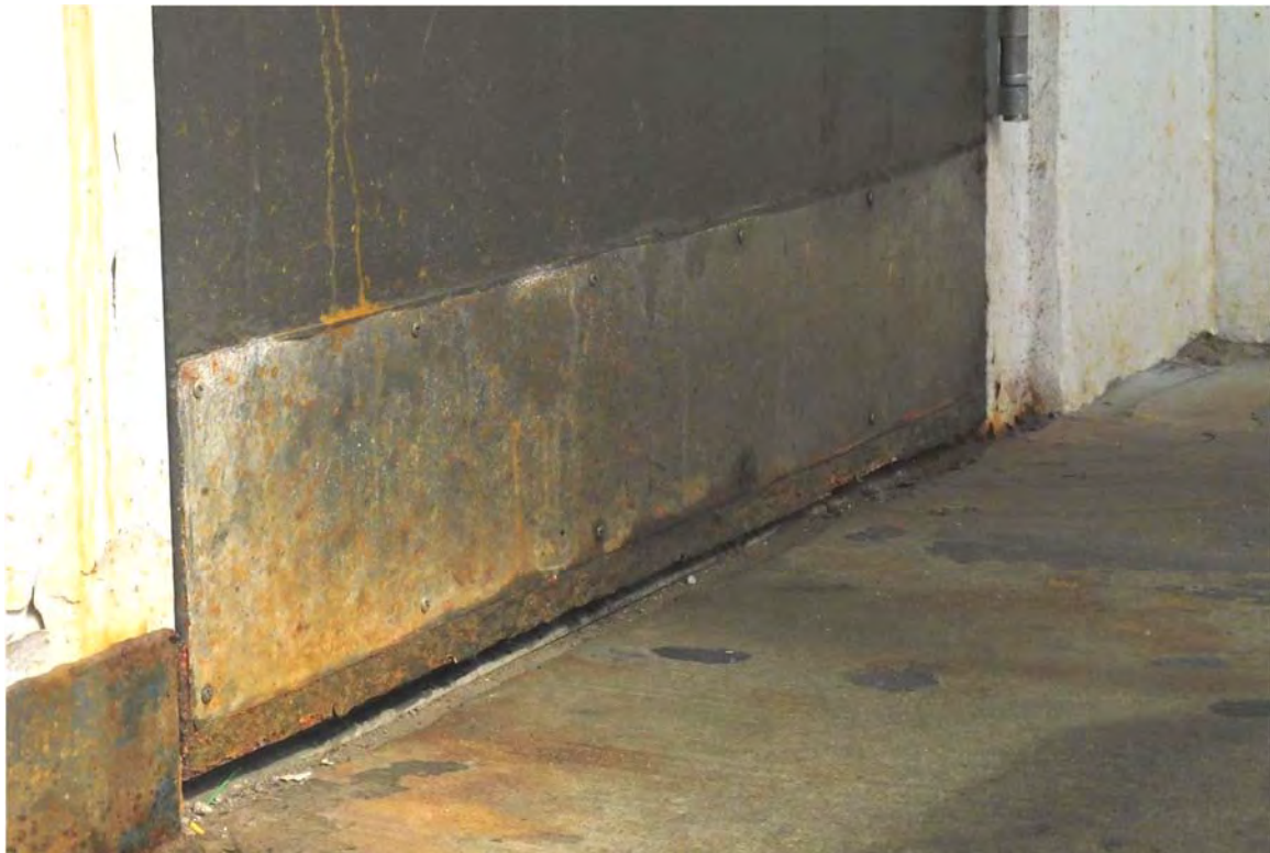
Photo 104 ...as well as the hollow metal doors was observed on each level of the southwest stair. Regular maintenance of the coatings on the doors and frames will help minimize the corrosion levels.
