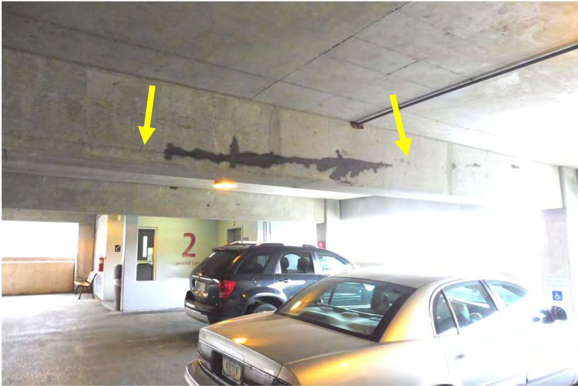
Photo 65 Level 3 beam seen from standing on Level 2 where grease from the tendons has leached out of the crack in the face of the beam.
