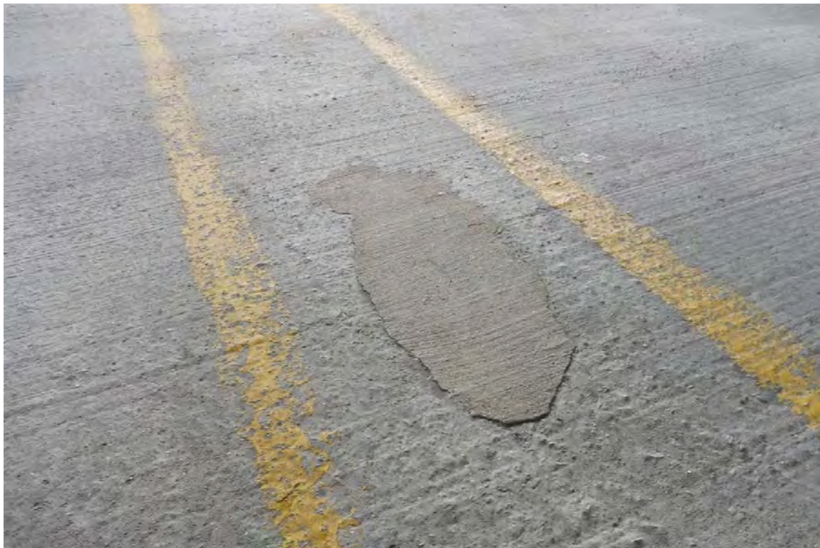
Photo 74 The floor slabs are in good condition while few existing patches were observed. The existing patch seen here was unsound and should be repaired.
