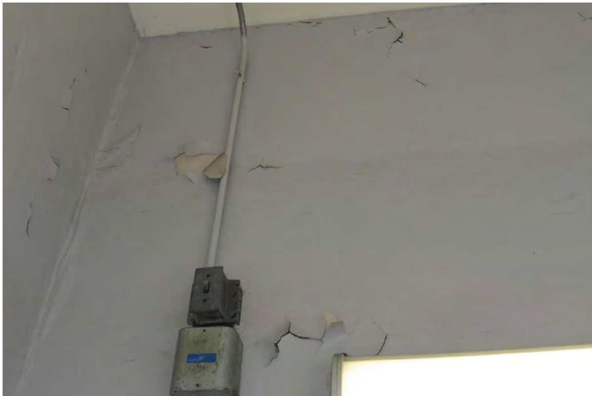
Photo 108 Example of the peeling and failed coating on the concrete walls within the southwest stair.
