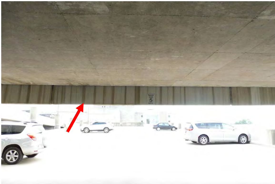
Photo 72 Staining on the back face of the edge spandrel is the result of water migration through the failed perimeter sealant joint above on the roof level.
