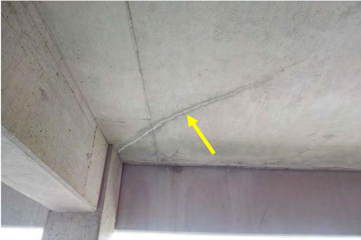
Photo 73 Cracks on the underside of the post-tensioned floor slabs existed in localized areas. The white staining seen along the crack is the result of calcium deposits on the surface from water migration through the crack.
