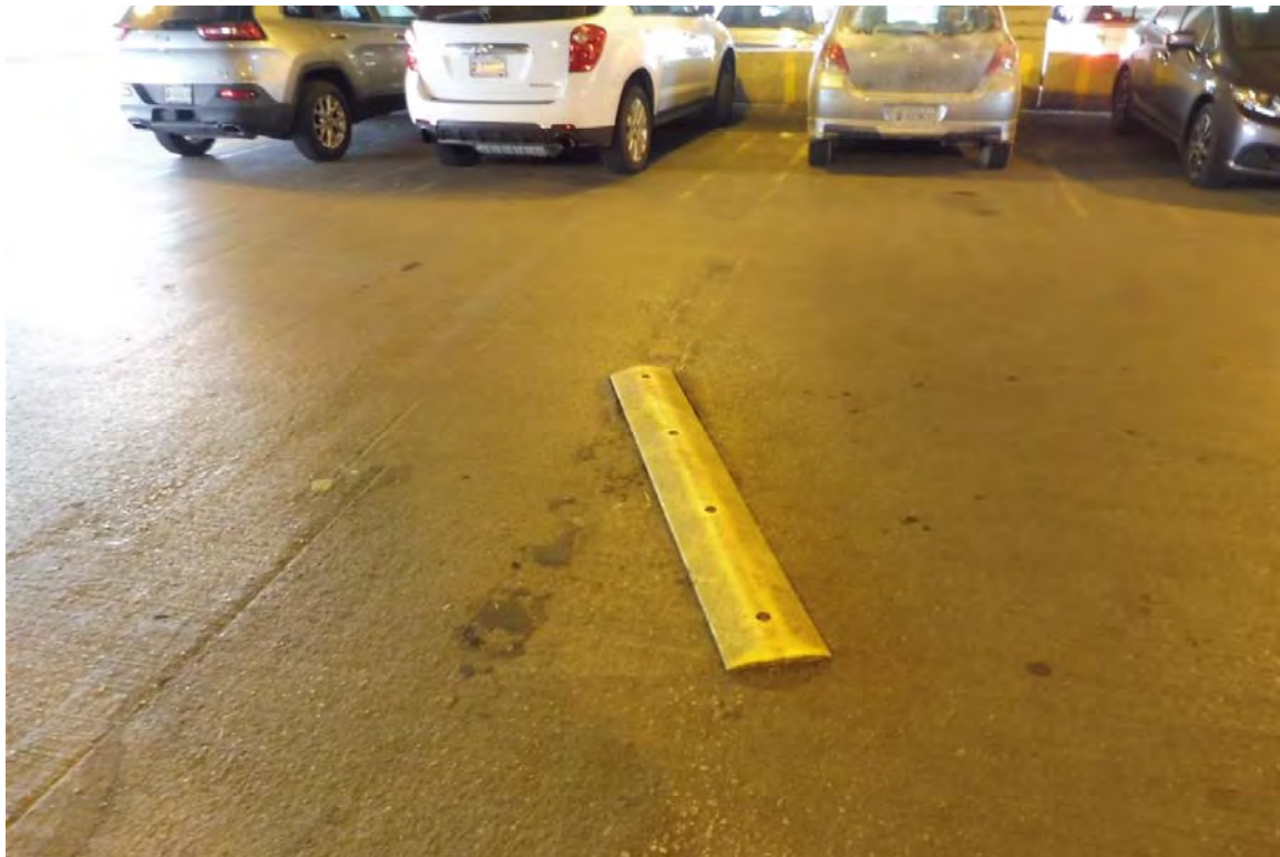
Photo 82 Speed bump devices have been installed. Several were missing and others were loose as seen here.
