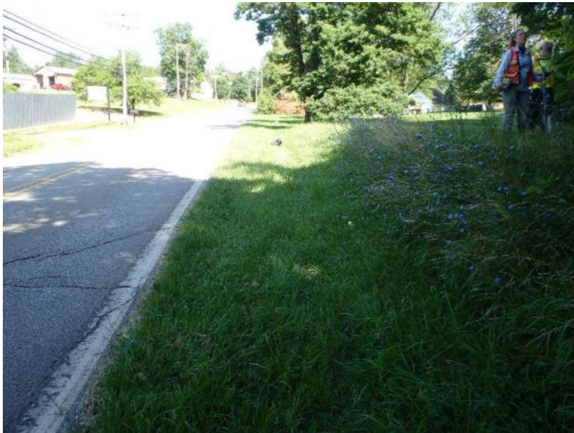
PP3 – Looking N at grassed side ditch along E Vernal Pike
