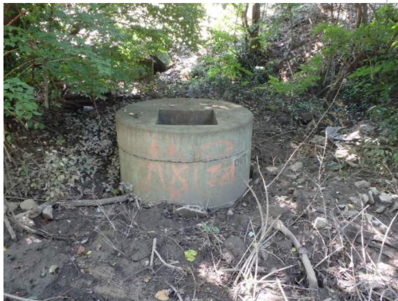
PP6 –Concrete stand pipe
