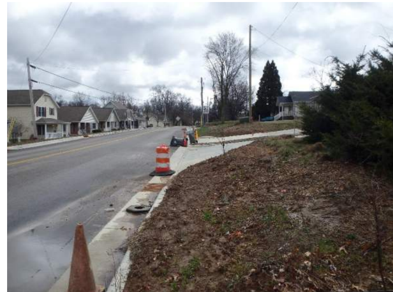
PP11 – Looking south along W Crescent
