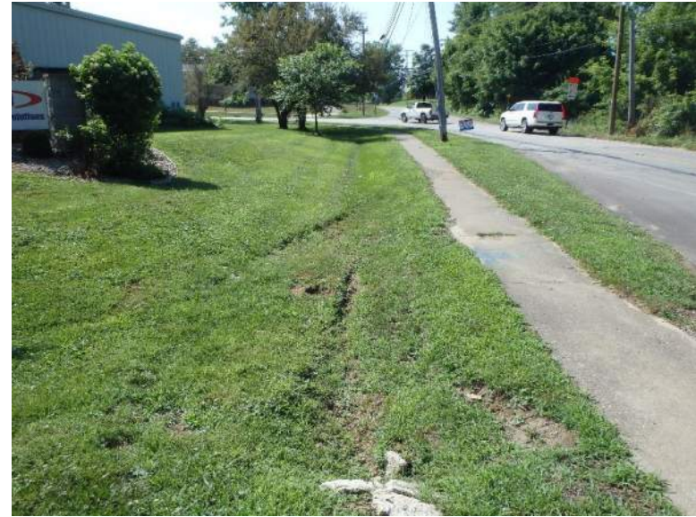
PP2 – Looking S at grassed side ditch along E Vernal Pike
