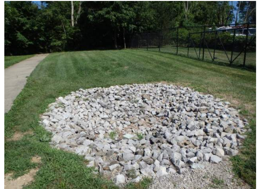
PP4 – Private property stormwater management feature
