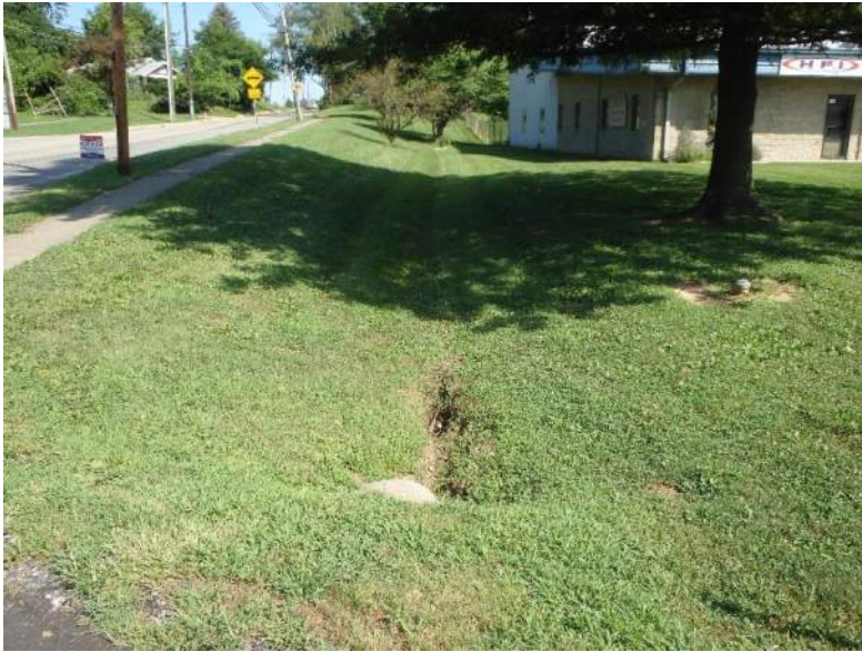
PP1 – Looking N at grassed side ditch along E Vernal Pike
