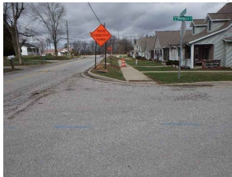
PP12 – looking north along E Crescent
