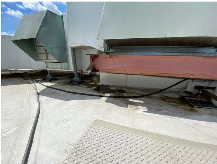
Main roof mechanical equipment condensation water ponding
