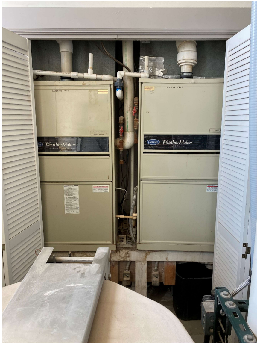
Furnace at first floor kiln room
