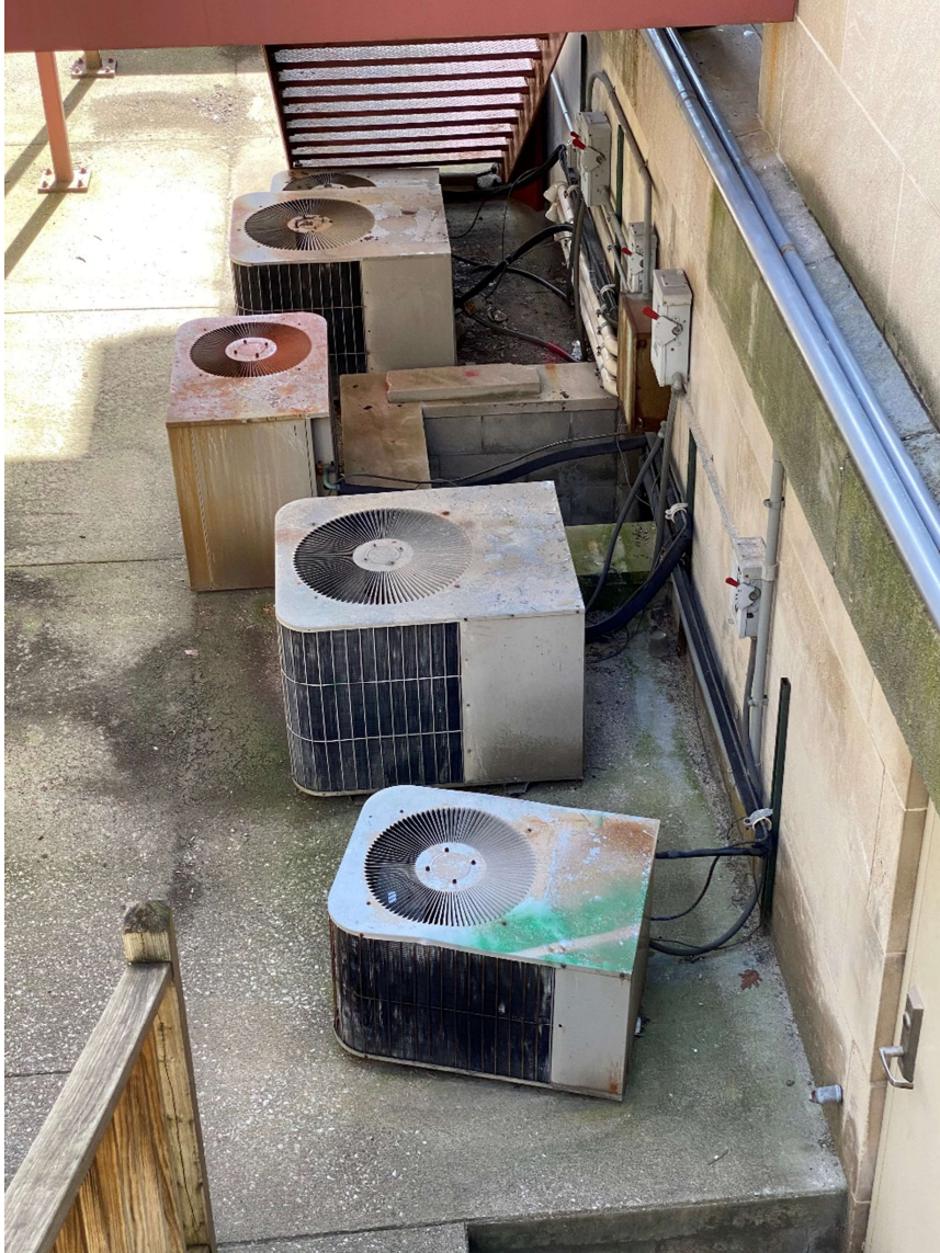
Old ACCU units at north exitway/alley enclosure
