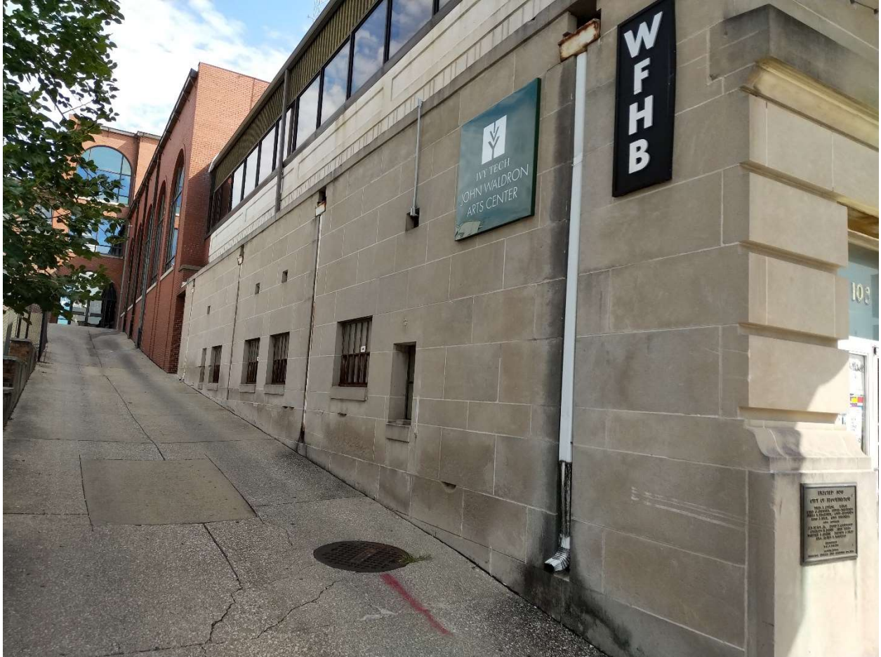
West alley exterior with issues in spalling, cracking, and drains.
