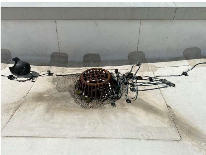
Main roof-roof drain debris
