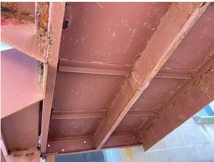
North exterior exit stair deterioration
