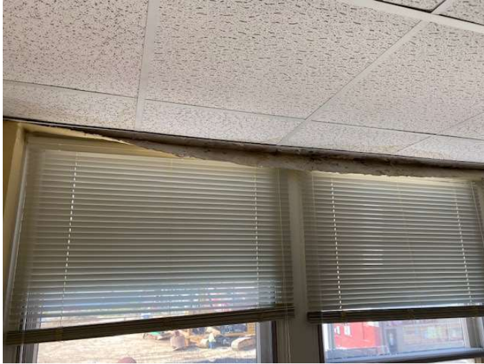
Second floor SW office window moisture issues
