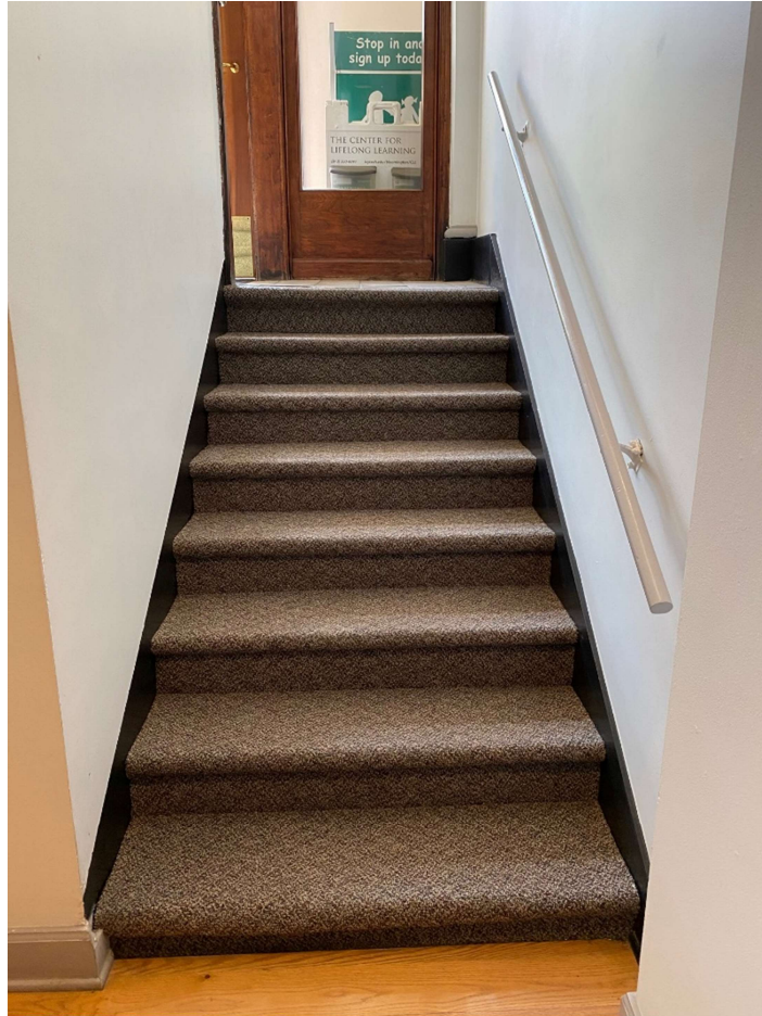
Typical stair railing-doesn't return to wall and not on both sides of stair
