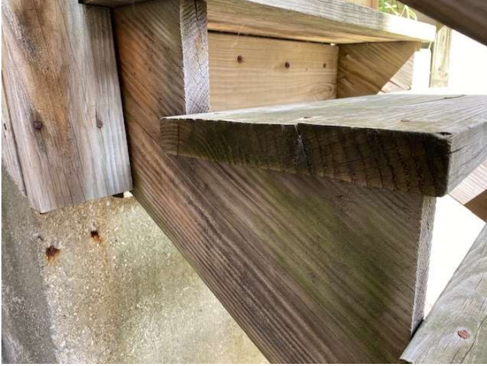
North wood exit stair rusted support fasteners
