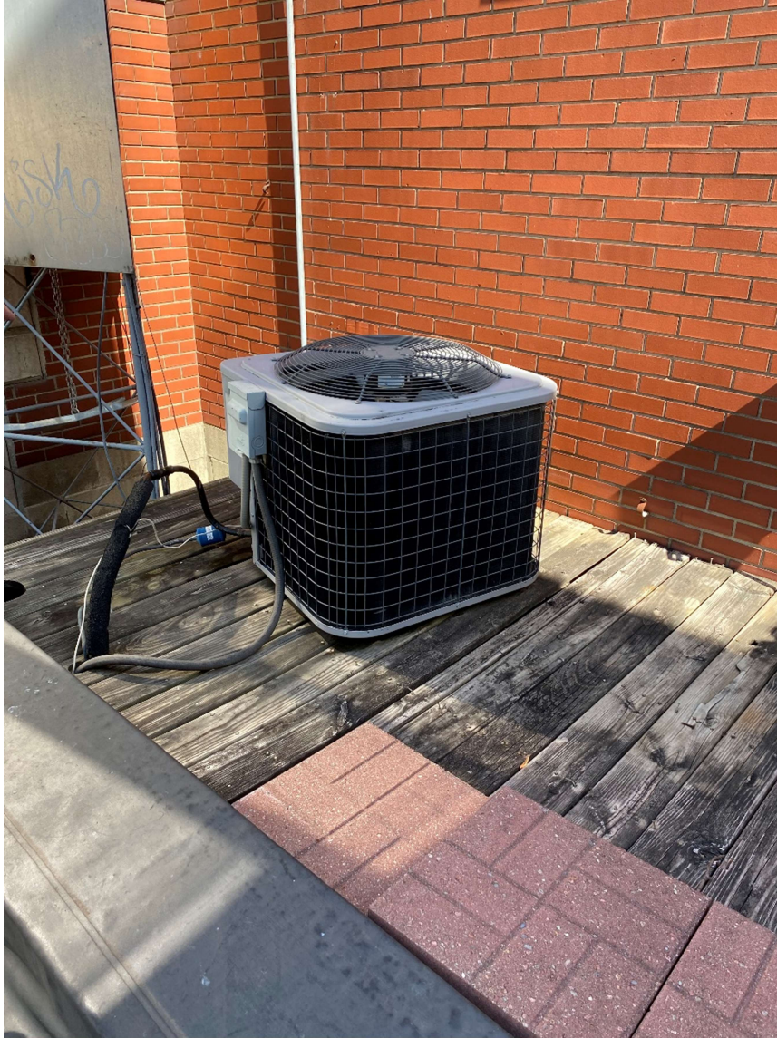
ACCU unit possible serving WFHB
