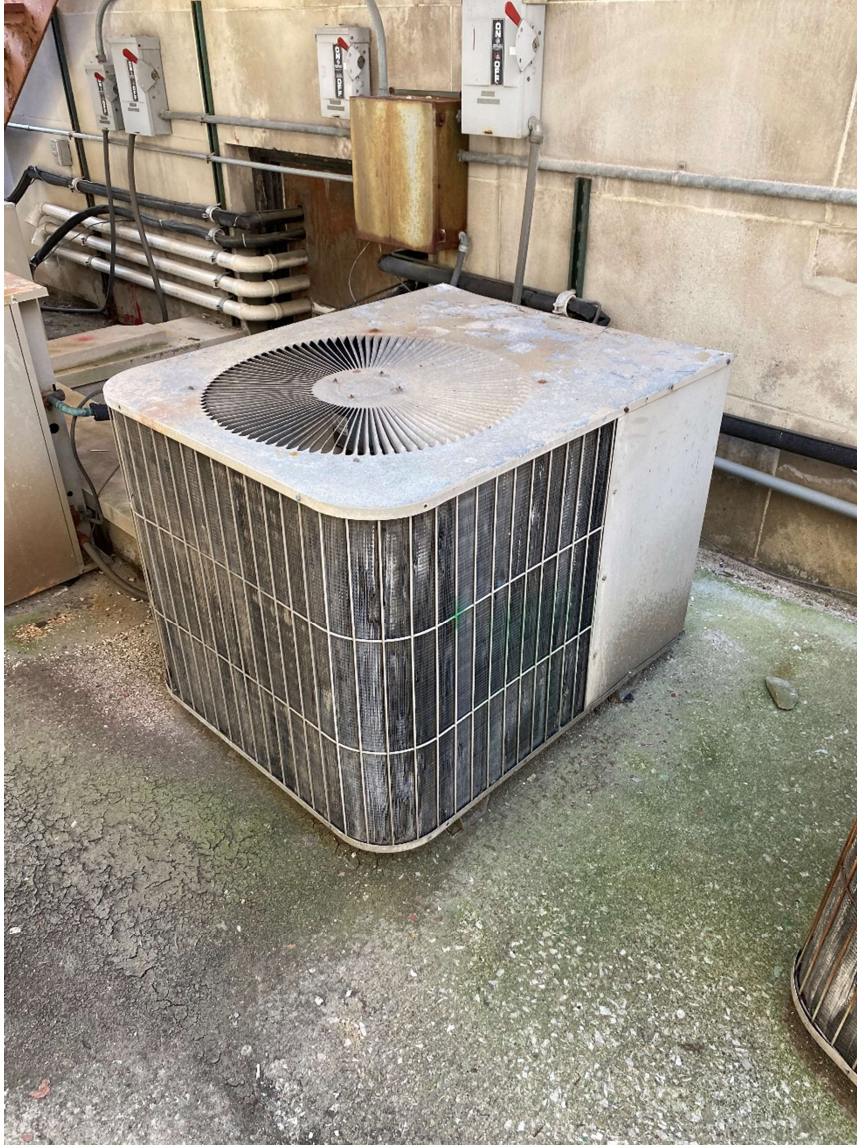
Failing ACCU in north alley/exit enclosure
