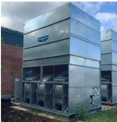
New cooling tower for the HVAC upgrade at City Hall
