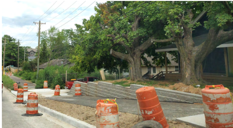
Multi-use path construction on Henderson Street
