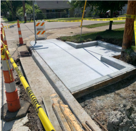
Bus stop improvement funded through Recover Forward
