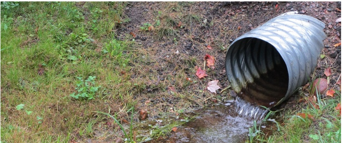
An Example of an Installed Driveway Culvert
