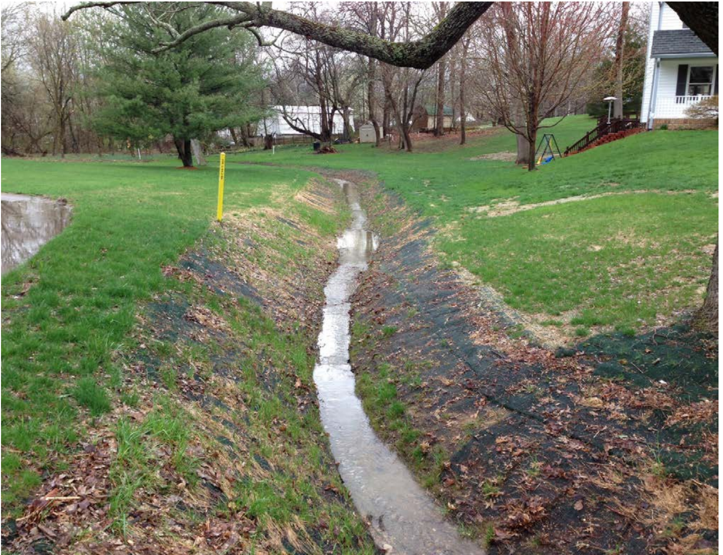
An example of ditch stabilization in progress
