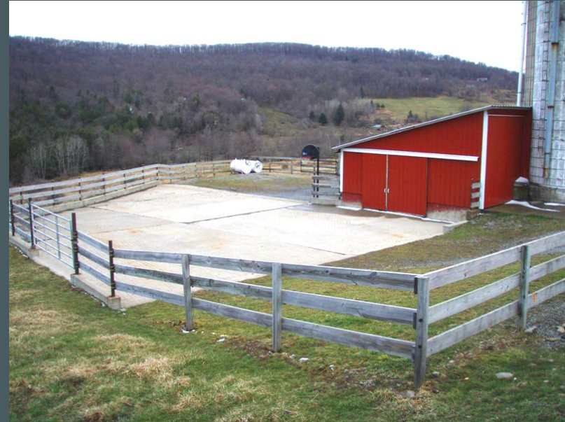
Stabilizing areas with heavy livestock usage.
