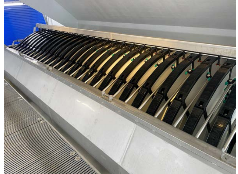
Disc filter at Dillman Road Wastewater Treatment Plant
