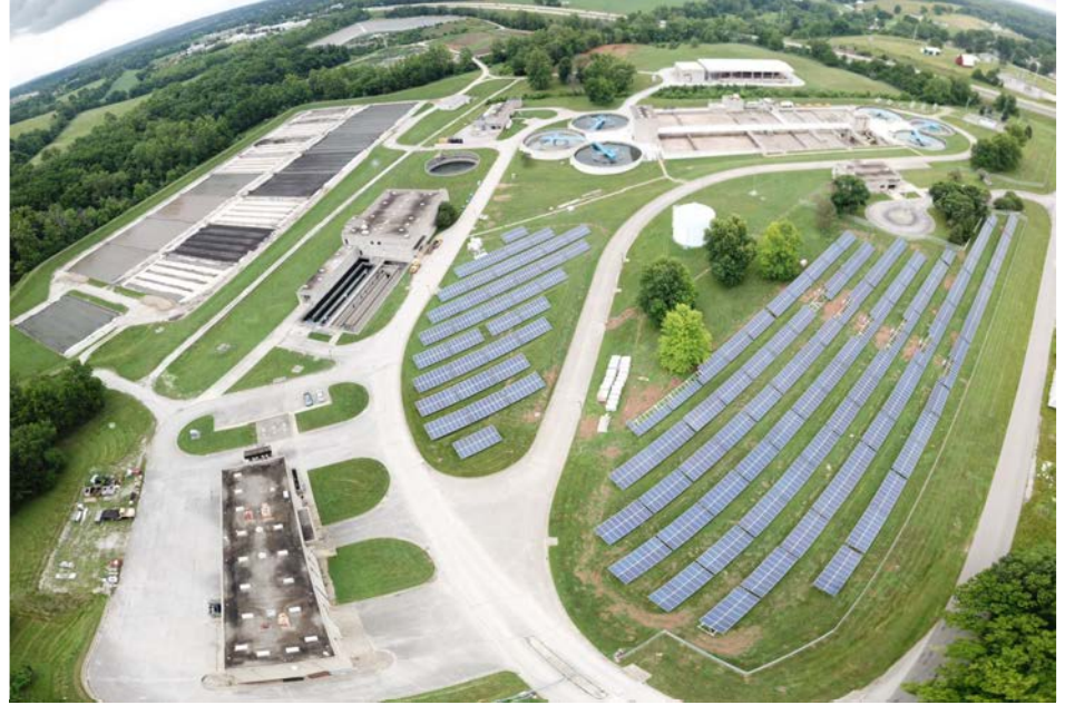
Solar panels at Dillman Road Wastewater Treatment Plant
