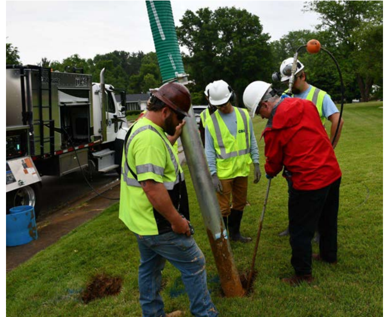
Mayor and crew working on Service Line Inventory
