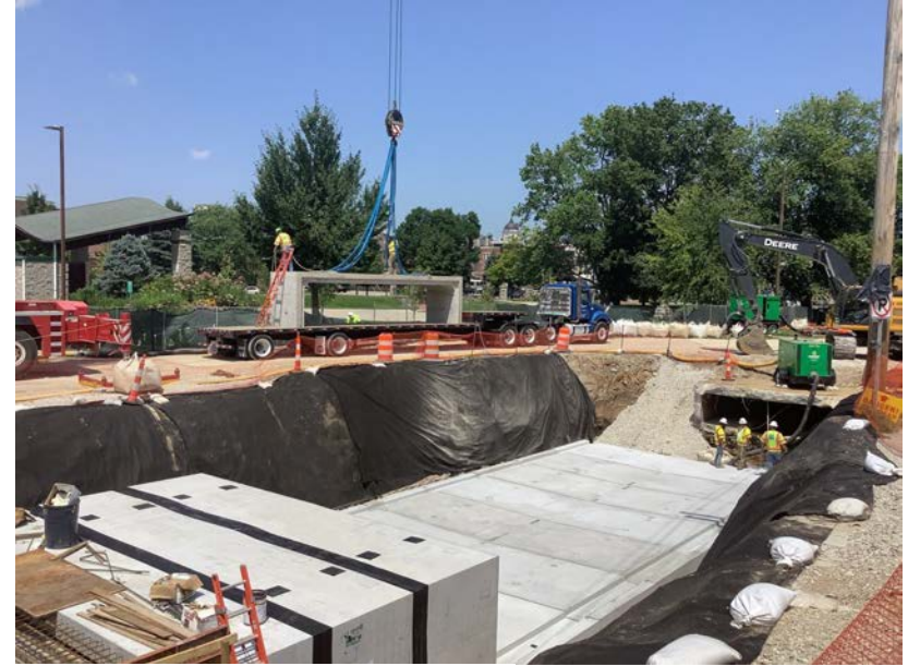
Hidden River culvert construction under Lincoln St
