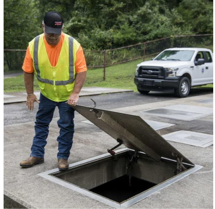
Checking Tammaron lift station
