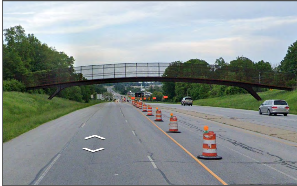
Pedestrian Bridge 45/46 Bypass
