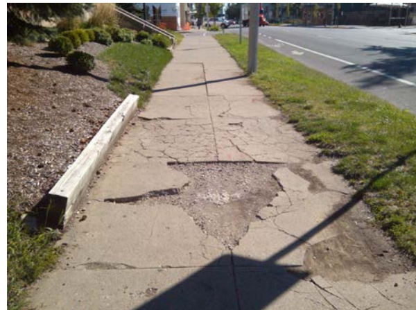
The ADA specifies that locations serving government facilities are given priority.
