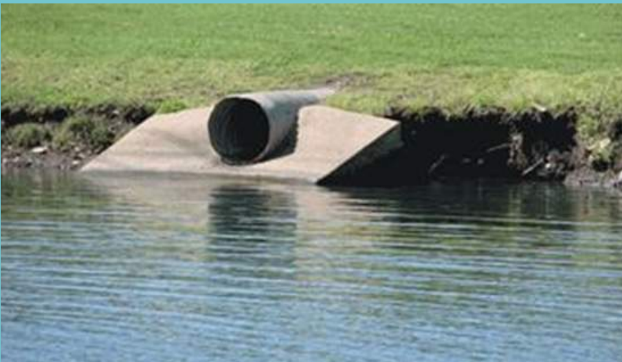
Wet detention pond
