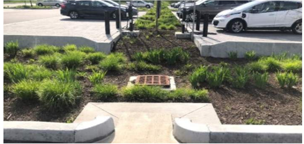
Bloomington, IN (Switchyard Park): Public parking lot using bioretention and permeable pavement to manage impervious surface and the stormwater runoff generated. Indianapolis, IN (Bioretention Bumpouts/Public R/W)
