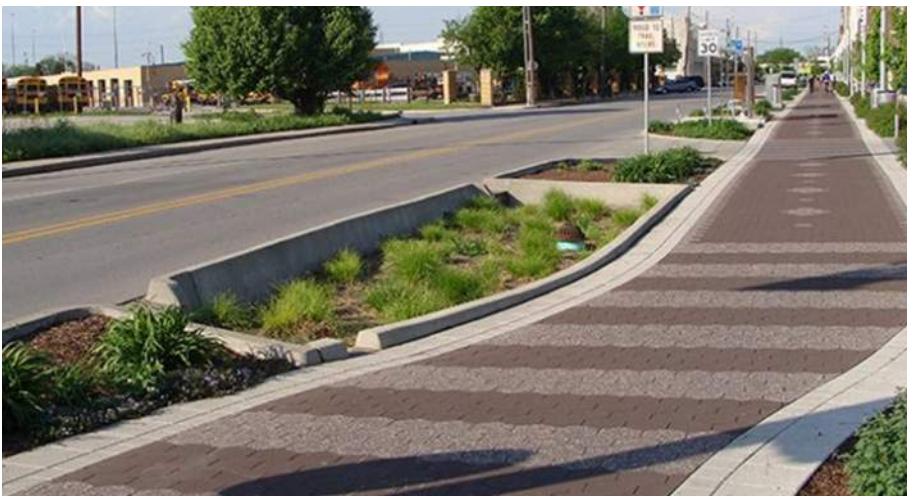
Indianapolis, IN (Cultural Trail): Bioretention bump outs in a R/W application to manage stormwater runoff from the street.
