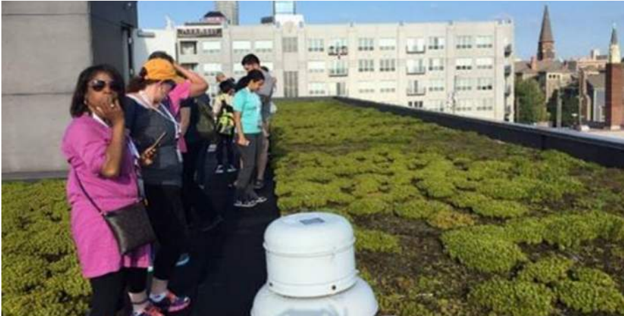
Indianapolis, IN (Nature Conservancy): Green roofs help minimize impervious surface and manage stormwater where it falls, while also providing an amenity on otherwise unused space.
