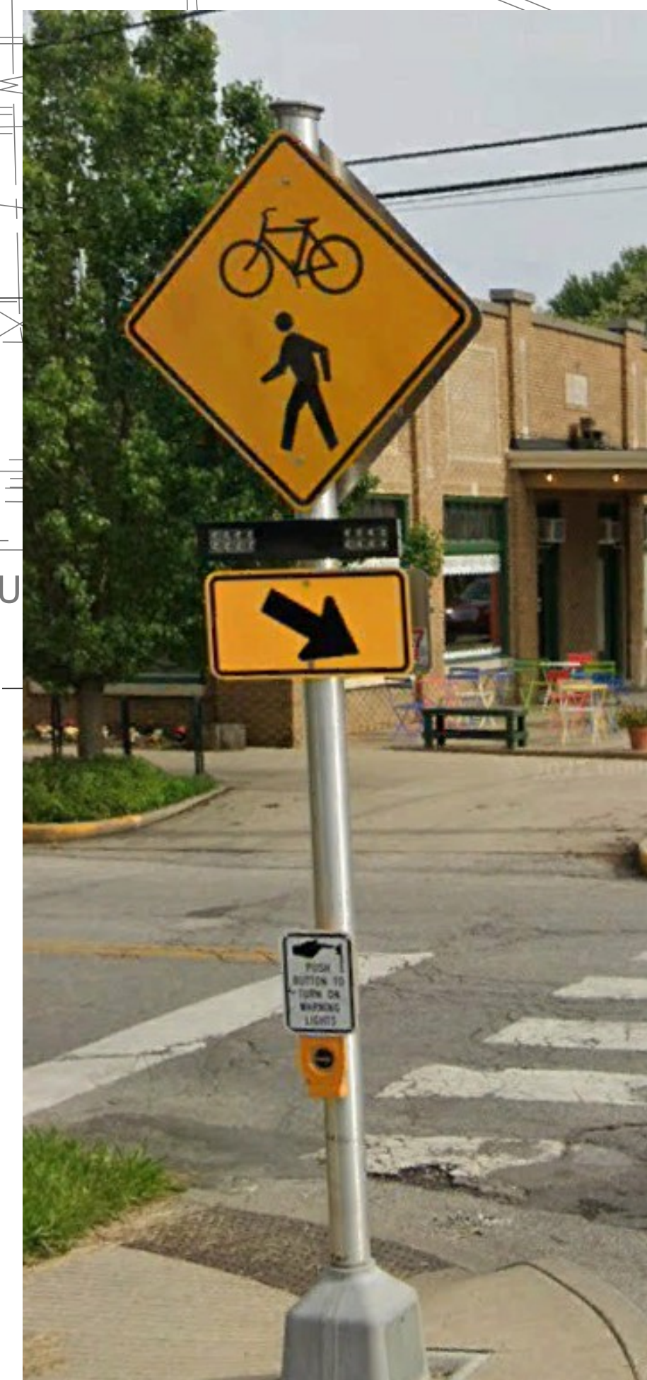
W11-15, W16-7p (Double-Sided) RRFB with Push Button Assembly
