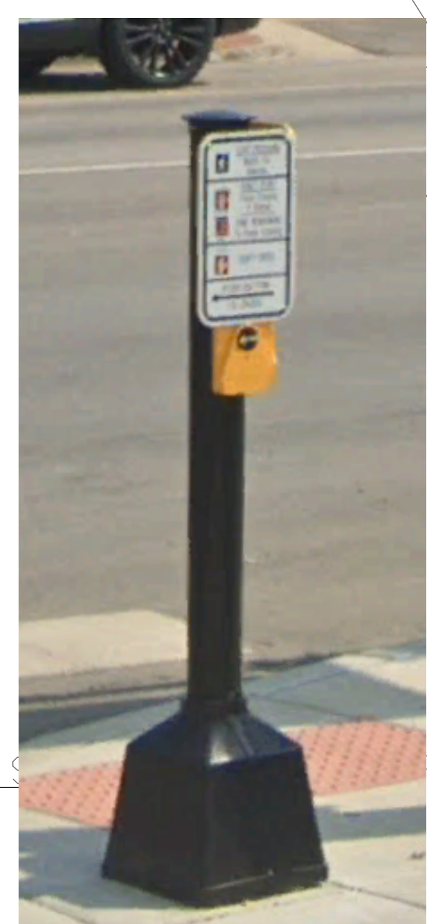
Pedestrian Push Button Assembly
