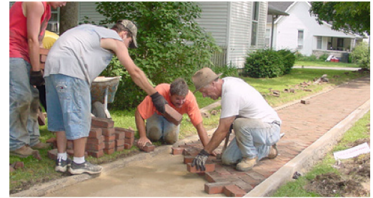
Bryan Park historic brick sidewalks restoration
