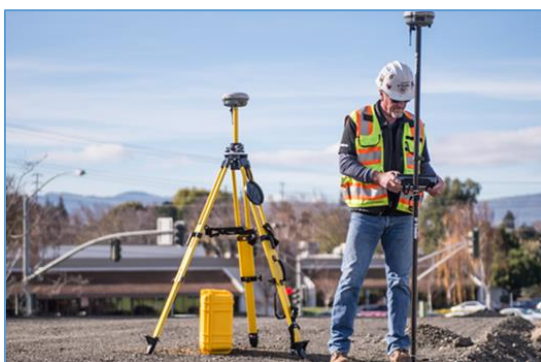
Mapping service lines with Trimble GPS and ArcGIS.
