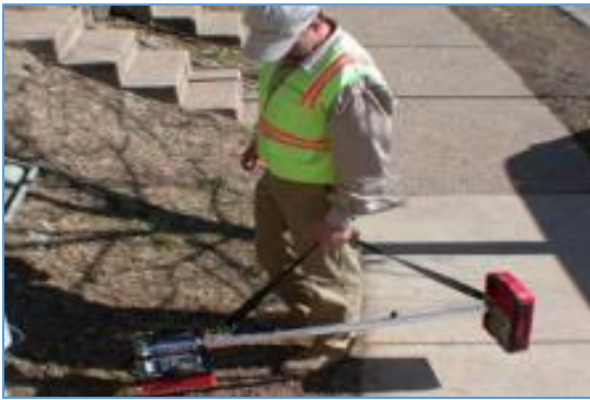
Line locating and painting.
