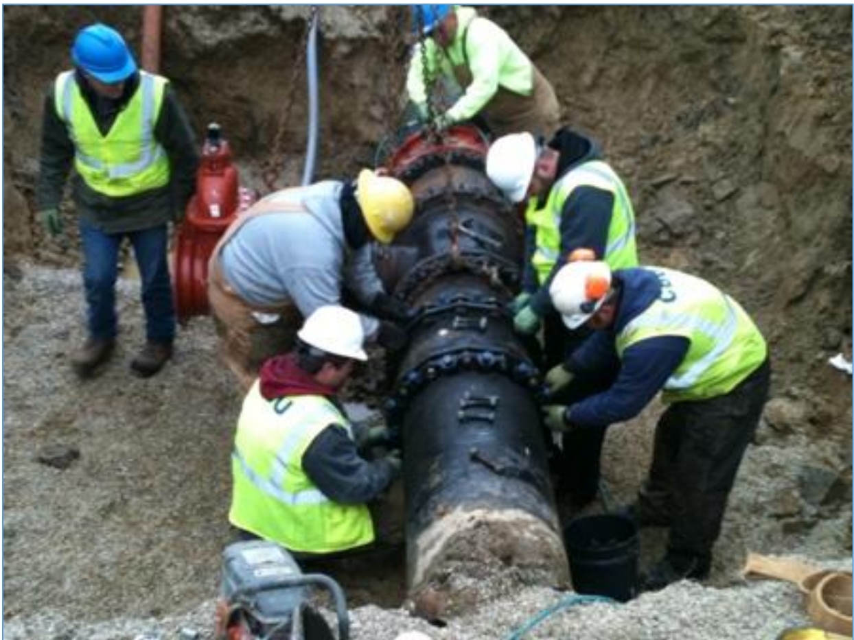
CBU water main installation.
