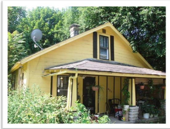
621 W 12th Street. Contributing. Architectural style: bungalow.
