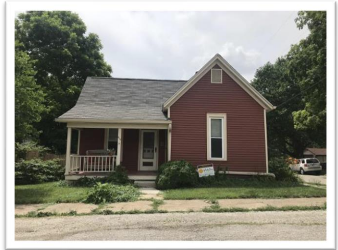
819 N Jackson Street. Contributing. Architectural style: gabled ell (c.1900).
