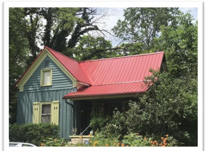
600 W 12th Street. Contributing. Architectural style: gabled ell (c. 1930).
