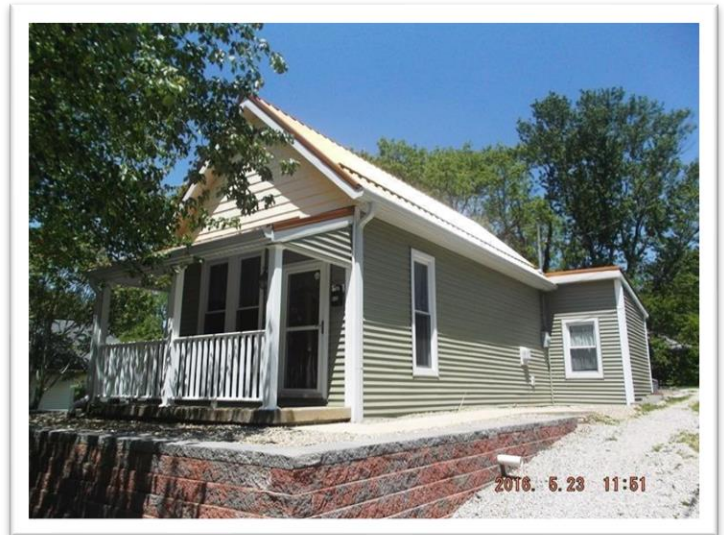
612 W 12th Street. Contributing. Architectural style: shotgun house.
